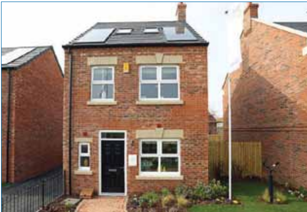
Farndale Housing Development
