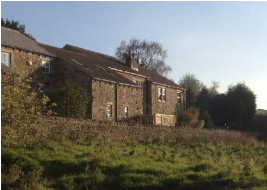
Above: The historic local vernacular interpreted successfully in modern development at Lidget Croft
