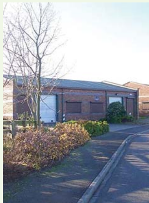
Workshop Units, Hinderwell
