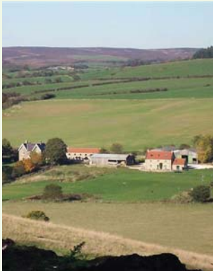
Agricultural Workers' Dwelling, Hardwick Farm, Harwood Dale
