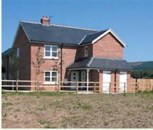
Affordable Housing, Battersby Junction
