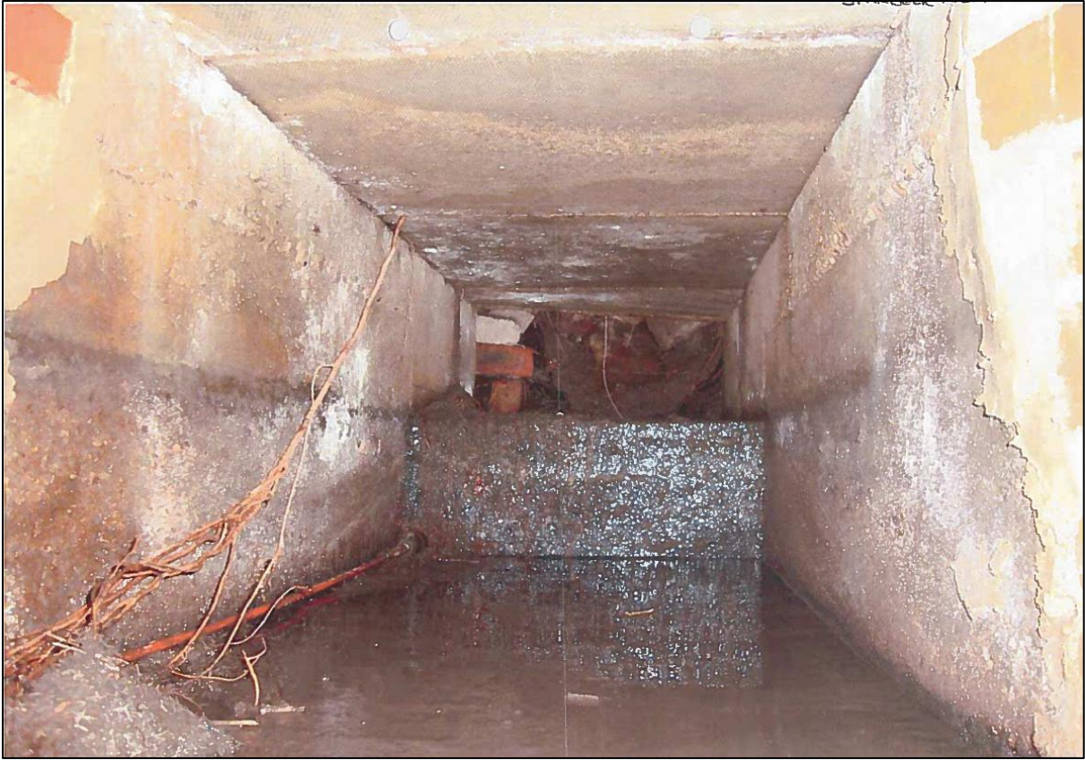
Figure 2.9 View upstream from Manhole at Hookstone Grange Way
