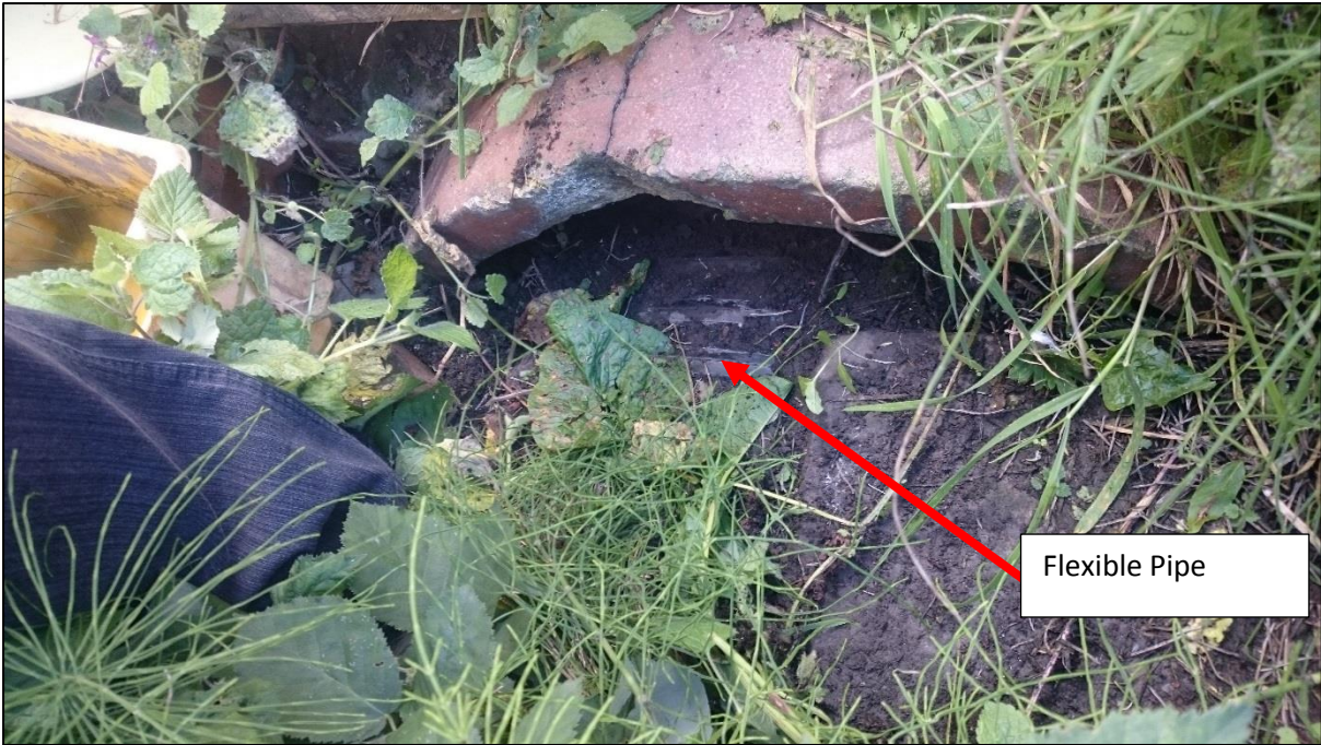
Figure 2.8 Connection between flexible pipe and culvert at 35 Greenfields Avenue
