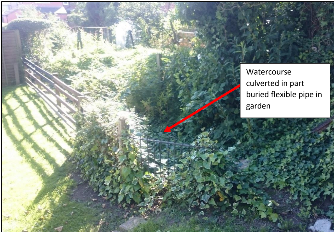
Figure 2.7 Flexible piped culvert
