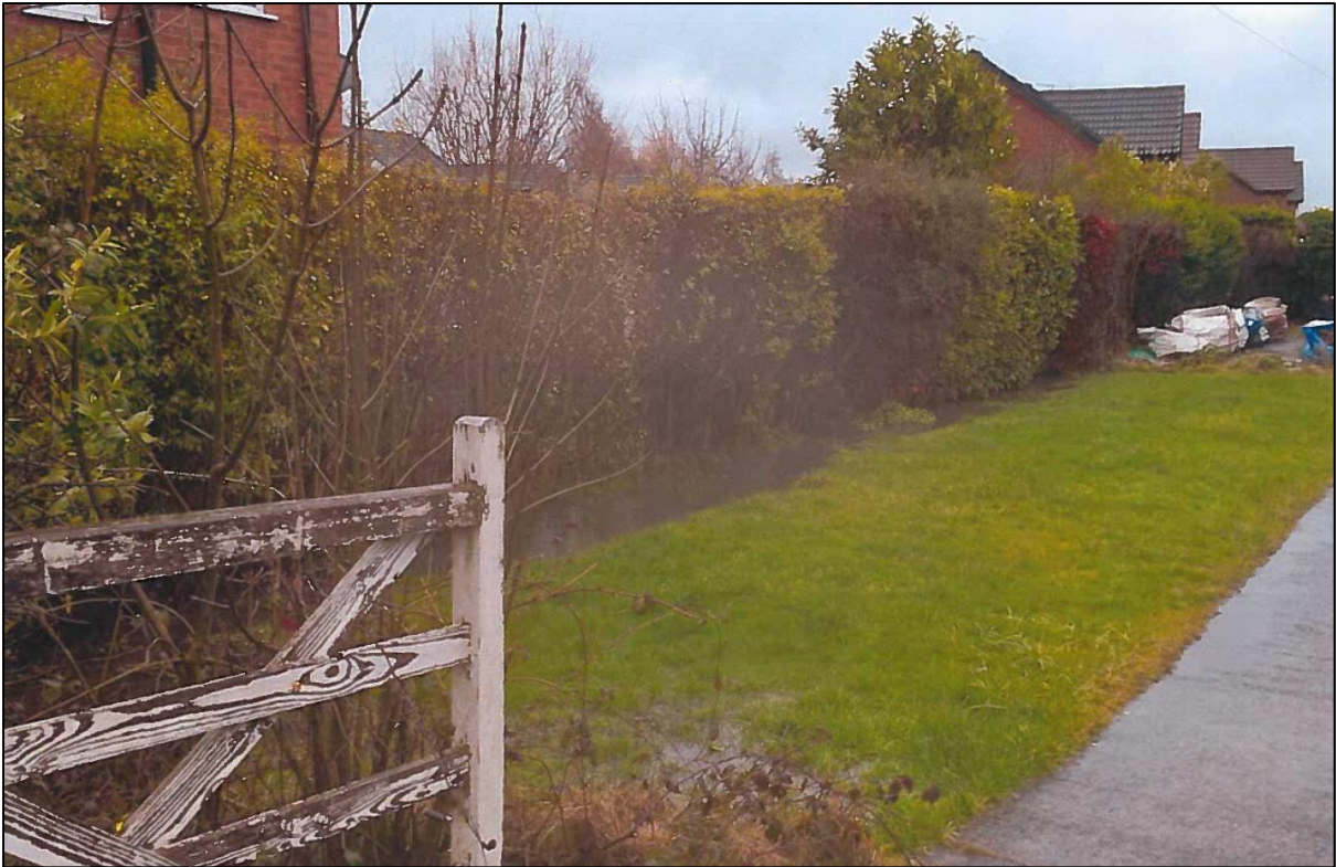
Figure 3.4 Photograph of flooding at Greenfields Avenue
