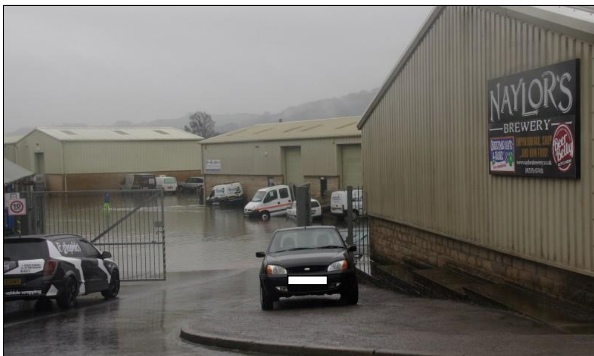
Figure 7.8 Photograph showing the flooding of Station Road Industrial Properties on Boxing Day 2015
