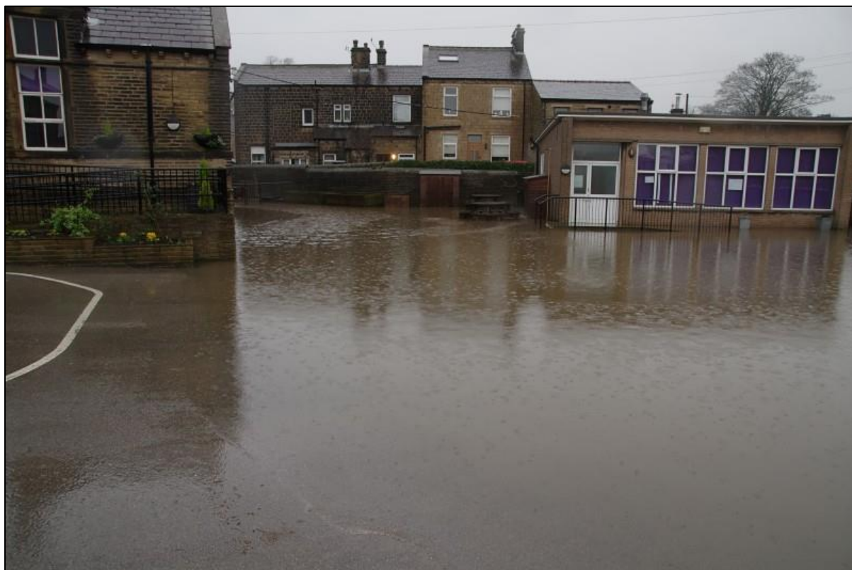
Figure 9.15 Photograph showing the ponding on the playground at the School
