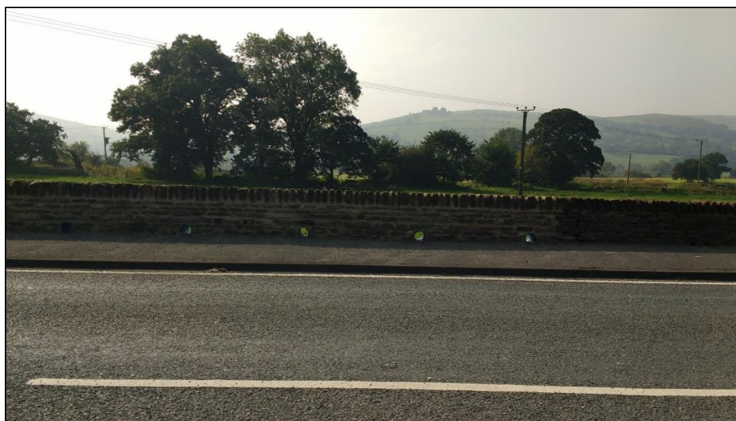
Figure 10.1 A629 at Ing Beck Bridge
