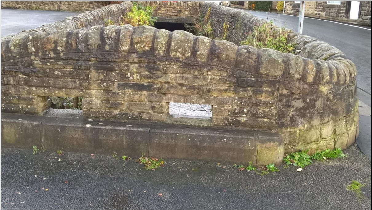
Figure 5.11 photograph showing Cononley Beck Bridge wall
