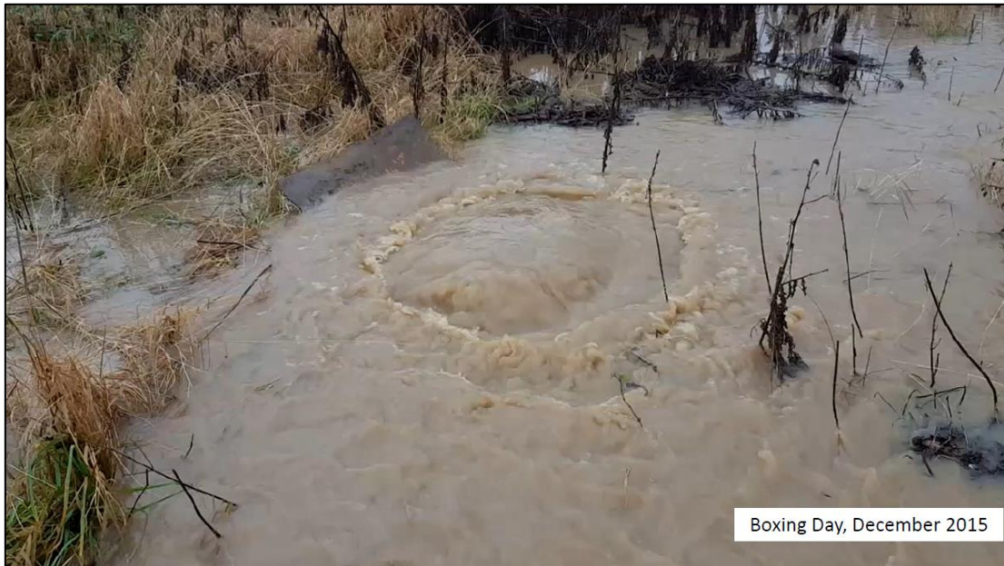
Figure 3.11 Photograph showing surface water discharge from manhole
