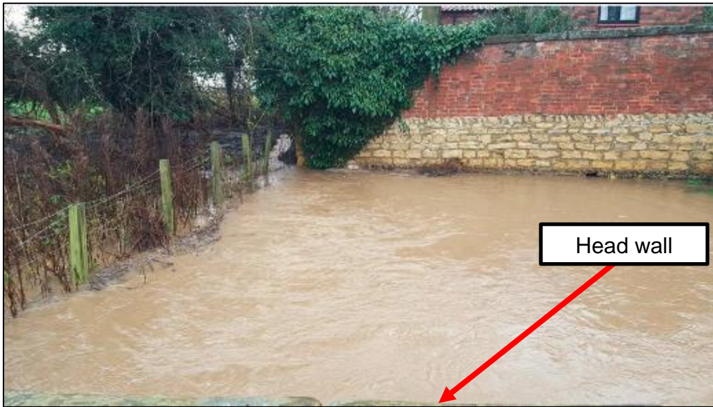
Figure 3.8 Photograph showing flood water behind headwall
