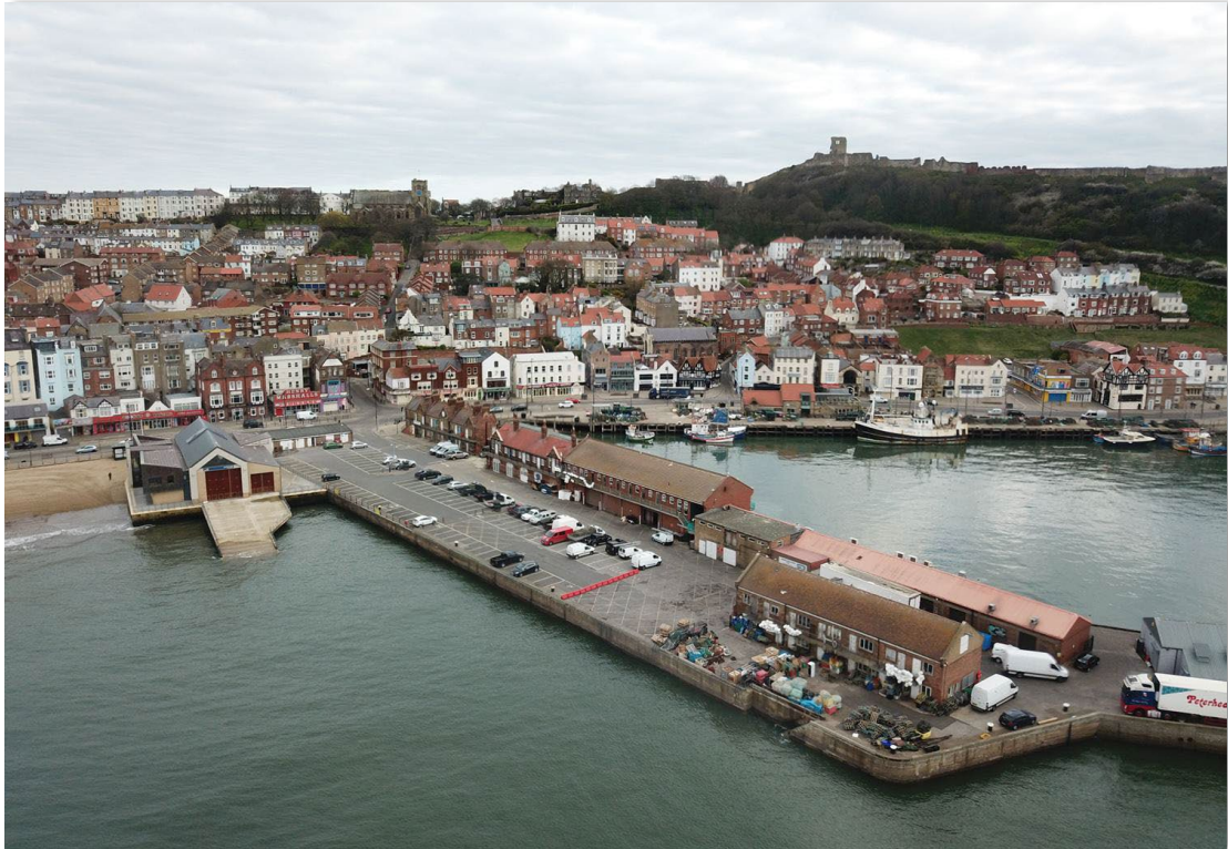
Image 1. Scarborough Harbour West Pier
