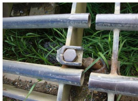
Longitudinal gap greater than 15mm
