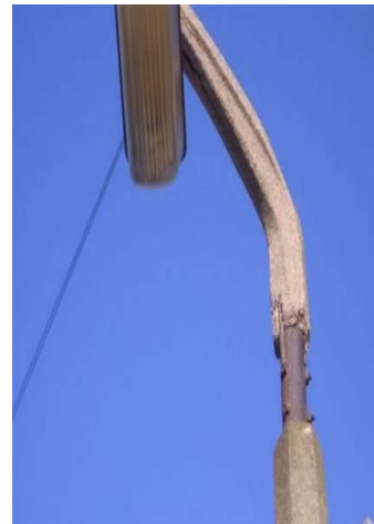
Spalling Concrete
