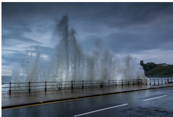
Climate change is increasing the risk of flooding and coastal erosion – Waves break over Marine Drive, Scarborough.
