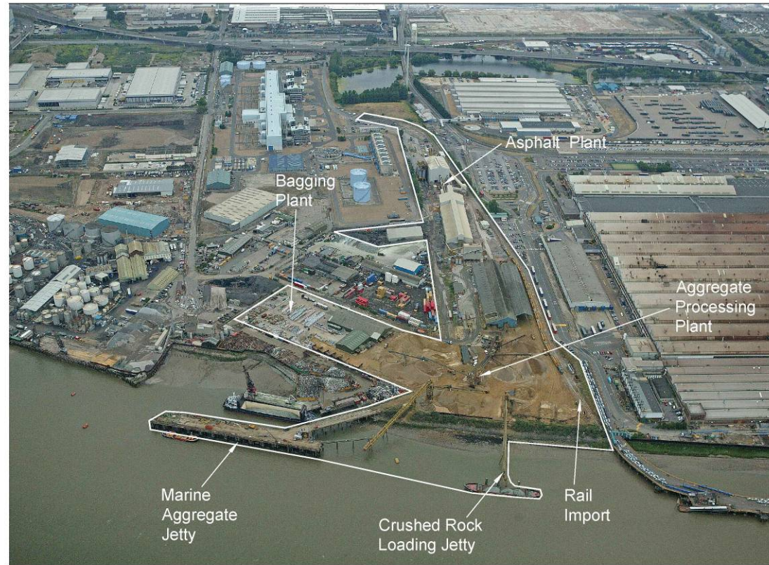
Photograph 9: Hanson UK Dagenham Marine Wharf and Rail Depot a large scale multi-modal facility on the Thames (courtesy of Hanson UK).
