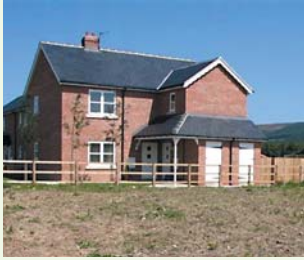
Affordable Housing, Battersby Junction
