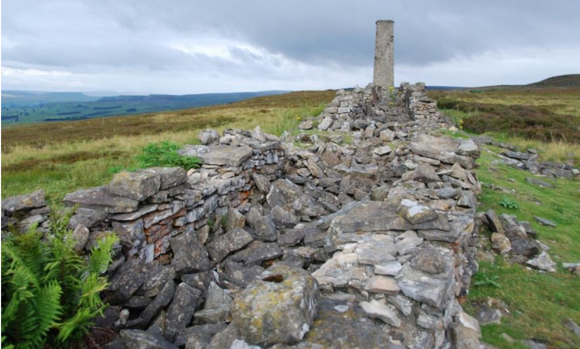
Figure 36: Cobscar Rake: Relict chimney and flue features associated with former lead mining activity on the ASMRP 14 limestone moors above Redmire Scar, in Wensleydale
