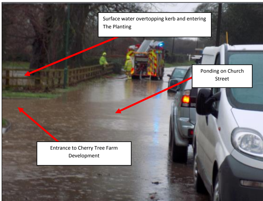
Figure 3.4 Photograph showing ponding on Church Street
