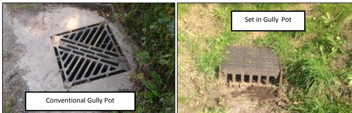
Figure 2.7 Church Street highway drainage gullies
