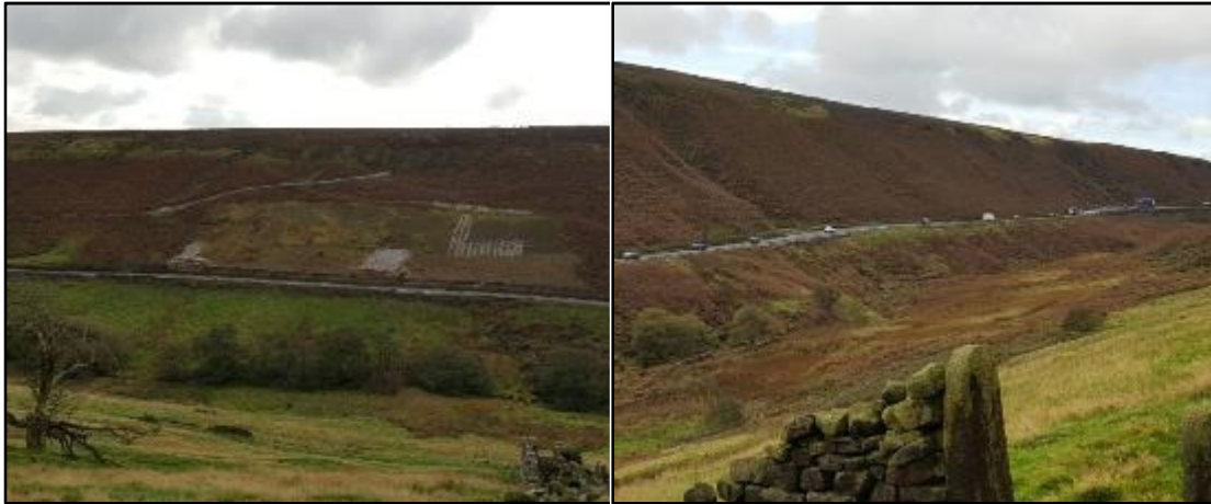
Kex Gill landslide area
