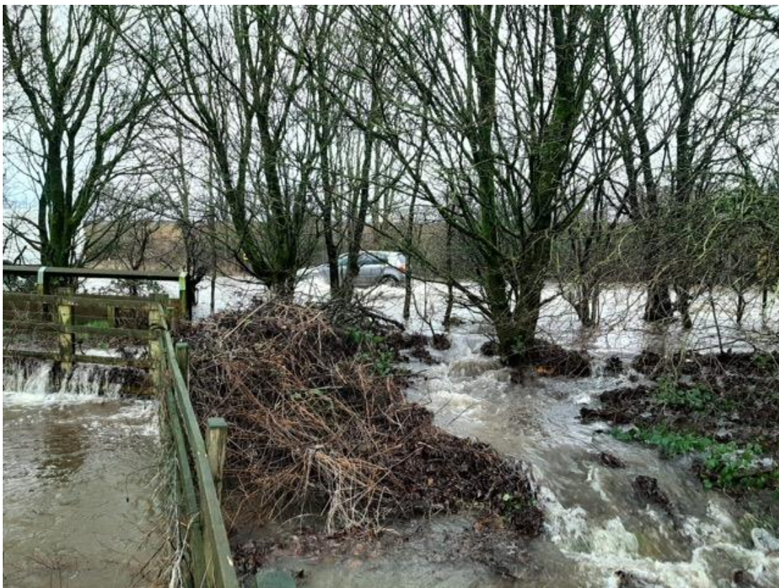
Figure 15: Gildersleets - floodwater by-passing bund
