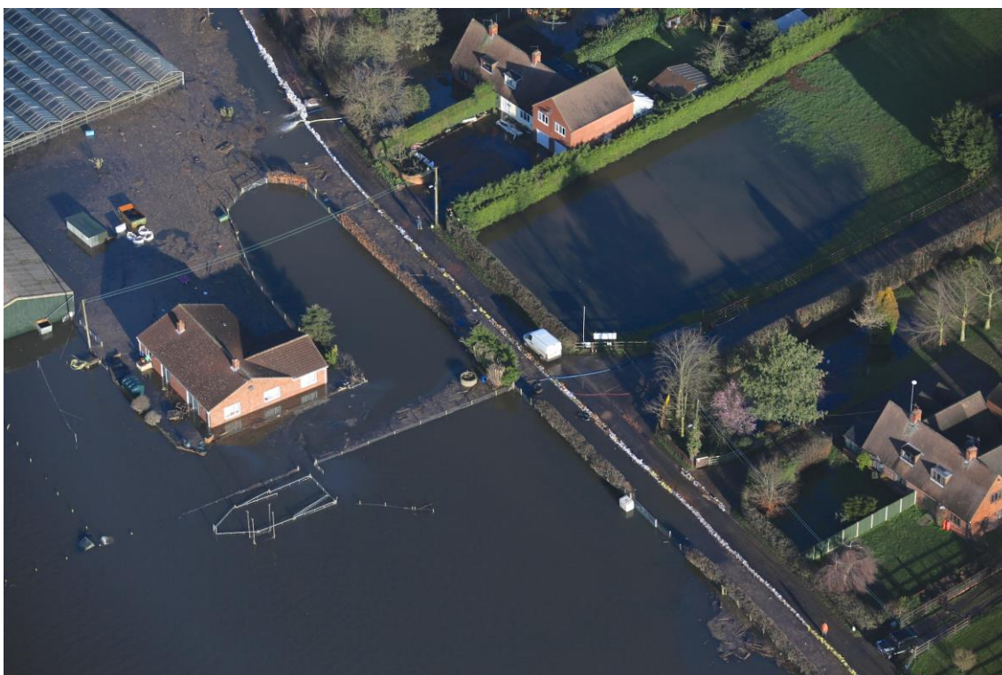
Figure 18: West Bank - Makeshift Defence
