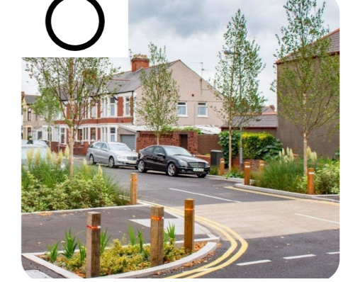
Speed reduction raised table with planted build outs to improve amenity.
