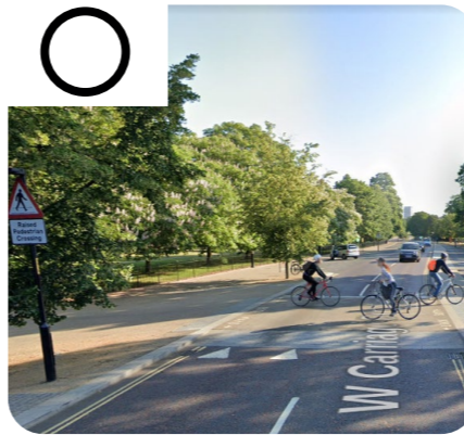
Speed reduction raised table with consistent surface treatment on all intersections along the route
