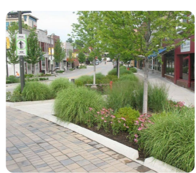
Rain gardens at junction build outs.
