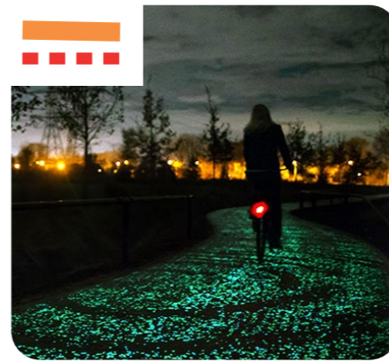
STARPATH technology to create wayfinding walkways - Spray on solution - Potential for use in combination with motion sensor street lighting along the corridor and links.
