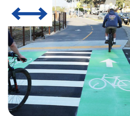
Zebra crossing raised zebra crossing with consistent colour surface to promote branding of Cinder Track
