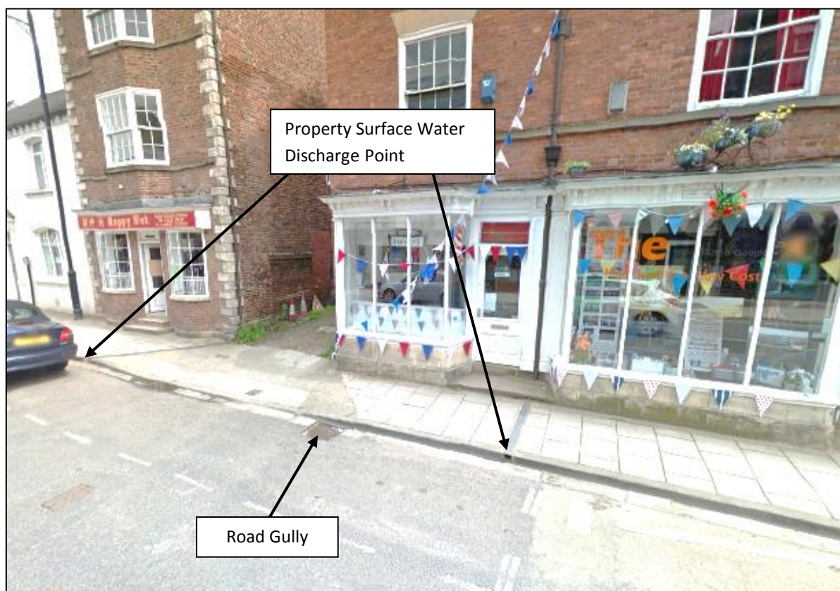
Figure 1.5 Bridge Street surface water components (Source: Google Maps)
