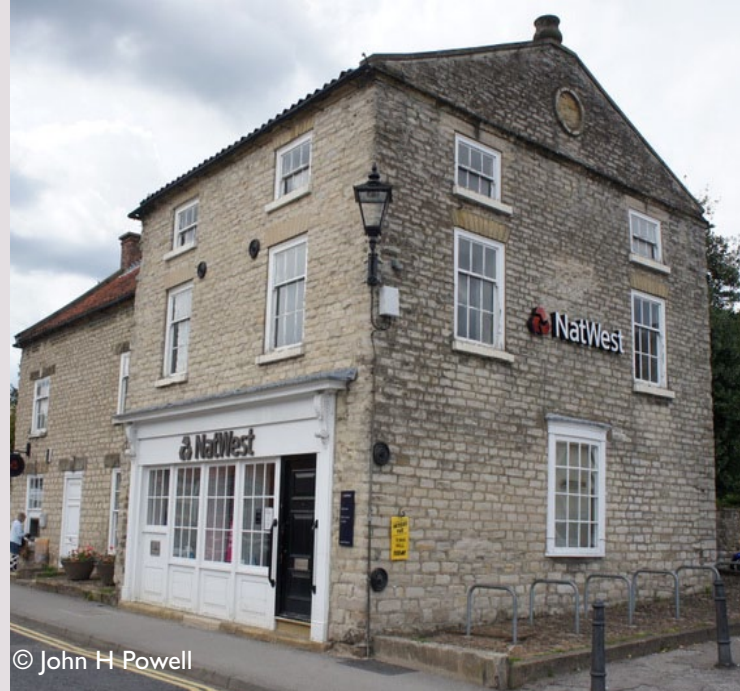
Above image shows pale-grey Hambleton Oolite Member used in a bank (former house) in Helmsley. Below image shows the use of Upper Jurassic Hildenley Limestone used in a finely carved arch at Kirkham Priory.
