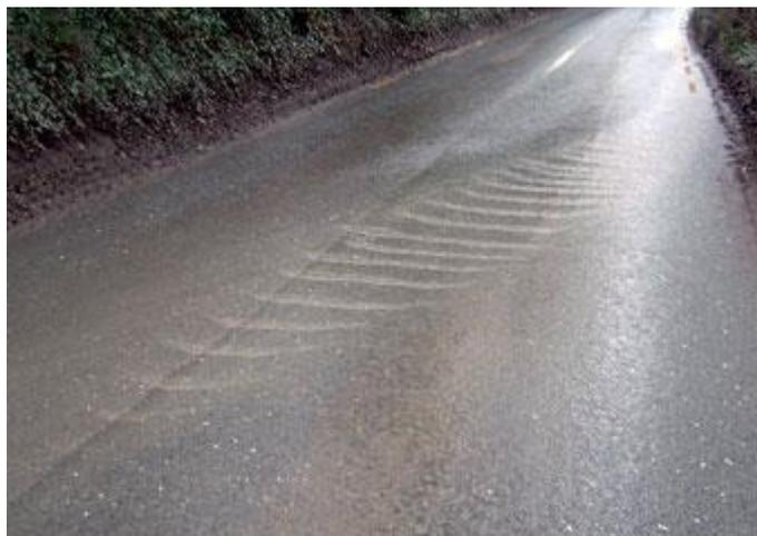
Water flowing across carriageway due to blocked highway drain
