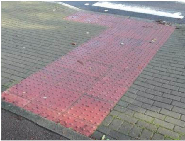
Figure 51 – Tactile Paving at a Controlled Crossing
