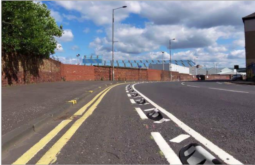
Figure 42 – Cycle Lane with Light Segregation
