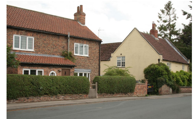
Low brick boundary walls and hedges on Church Street. This image also shows a probable former thatched cottage (number 3 Church Street) of possible 17th century date.
