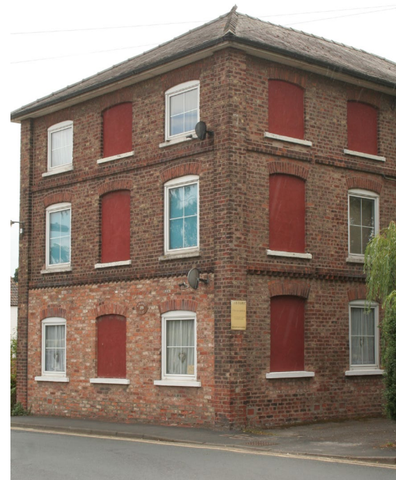
39 Main Street, a possible 19th century industrial building. Note the blind central windows and the Welsh slate roof.
