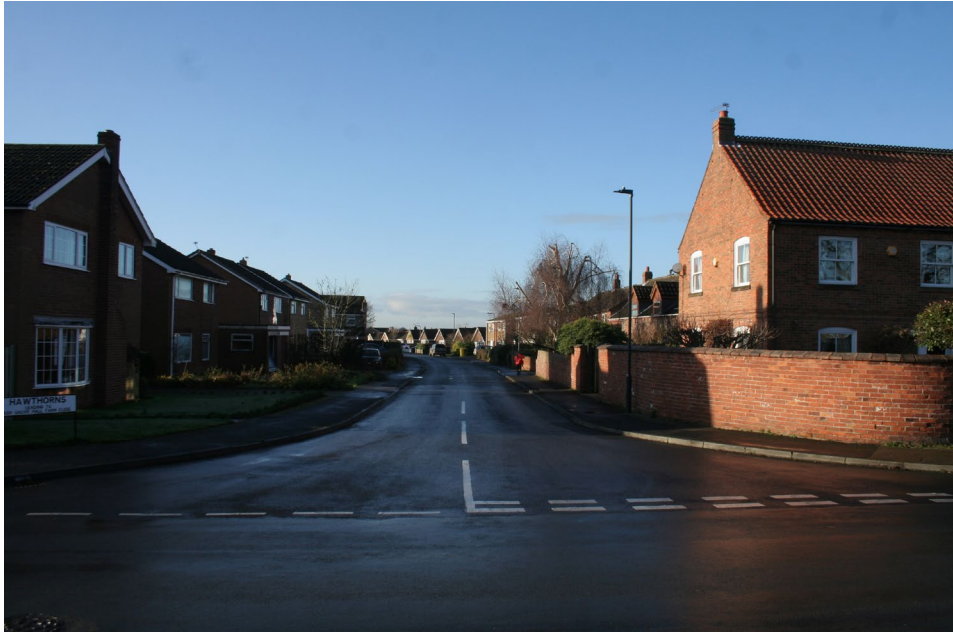
View of late 20th century housing on Hawthorns looking west from Church Street. Note the slayed junction and rebuilt brick wall to the right.
