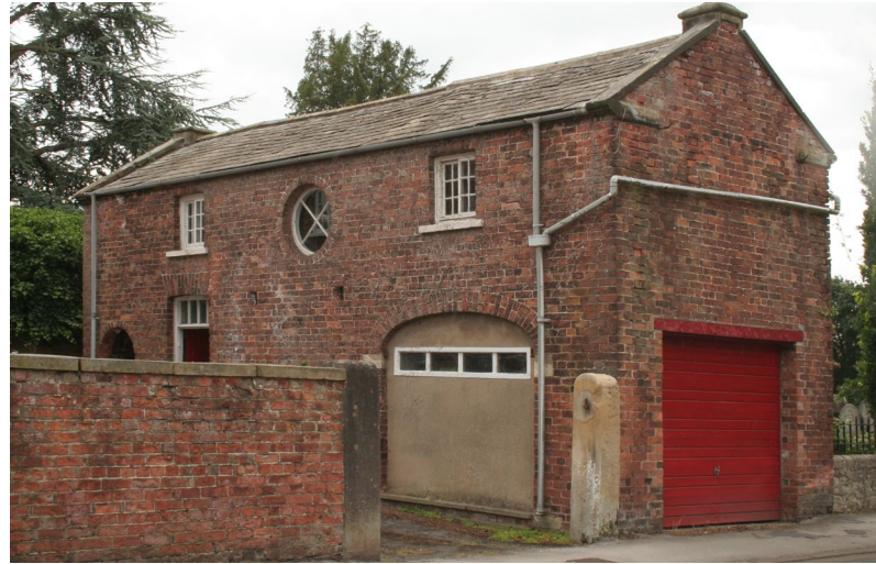
The Grade II listed Red House outbuilding. Note the Welsh slate roof.
