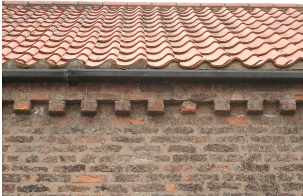
Roof detail, hand made brick and replacement clay pantile roof
