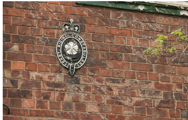
Late 19th century machine made brick with police house plaque on Main Street
