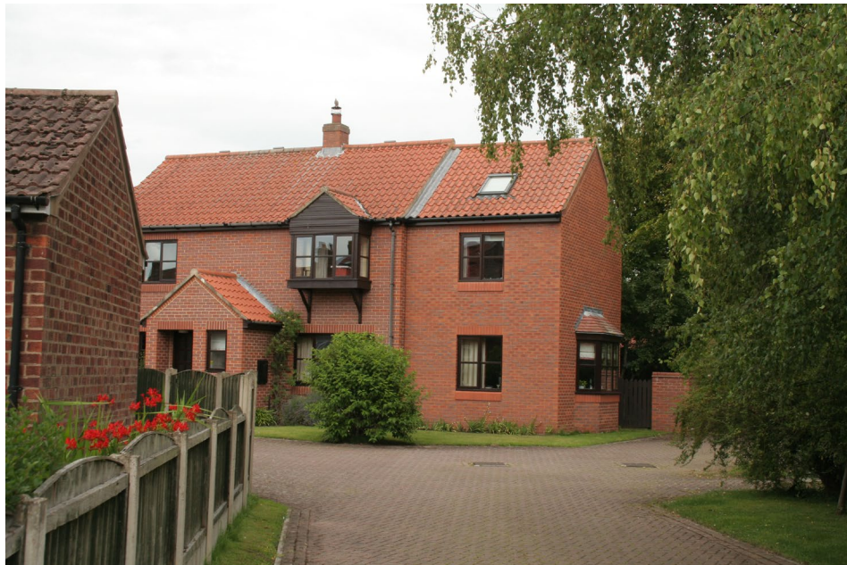
Late 20th century housing to the rear of 30 Main Street. Note the intrusive block paving and property design.
