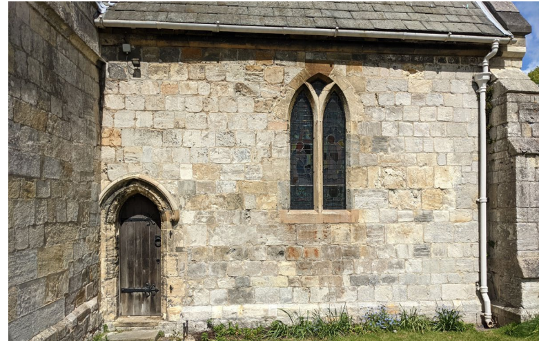
Close up of the 13th century chancel showing one of the lancet windows and contemporary doorway.
