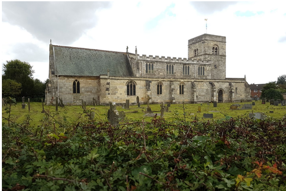
St Mary's Church from Silver Street showing 12th century tower and 13th century chancel
