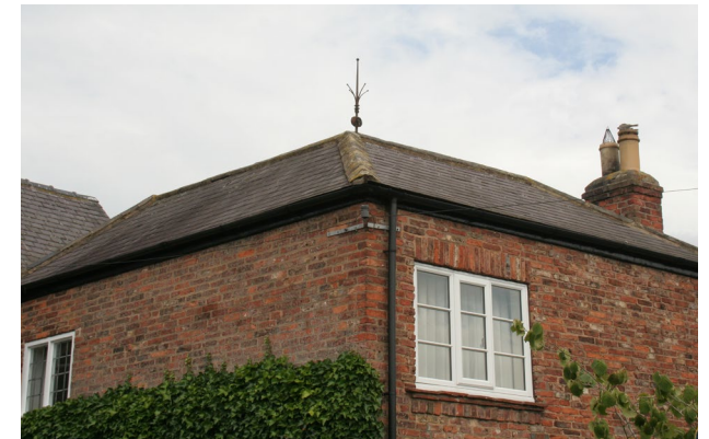
Welsh Slate and other roof detail on 44 Main Street
