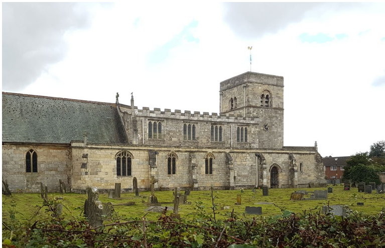
Magnesian limestone construction on the Grade I listed St Mary's Church. Note the Welsh slate chancel roof.
