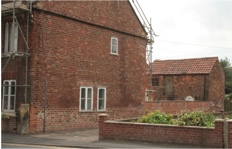
Outbuildings to the rear of 33 Main Street. Note the clay pantiles.
