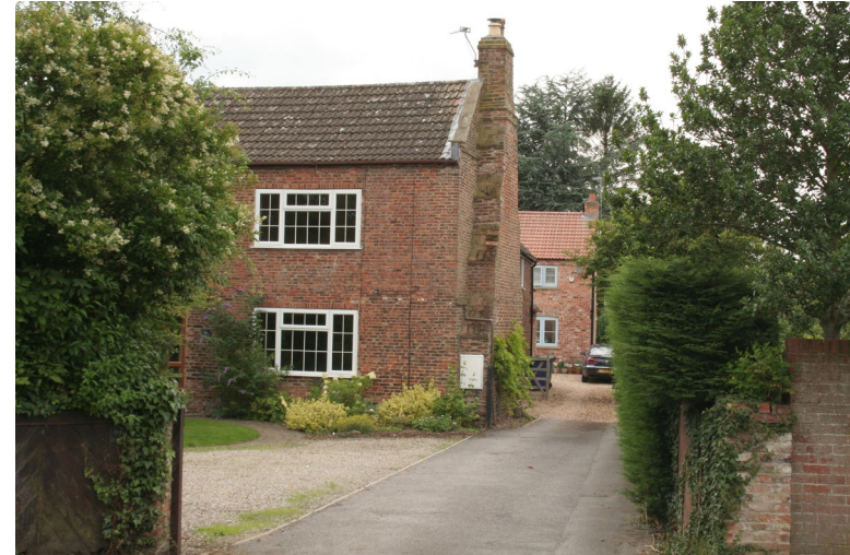
Reconstituted stone pantiles and uPVC windows on an early to mid 19th century former farmhouse (8 Church Street)
