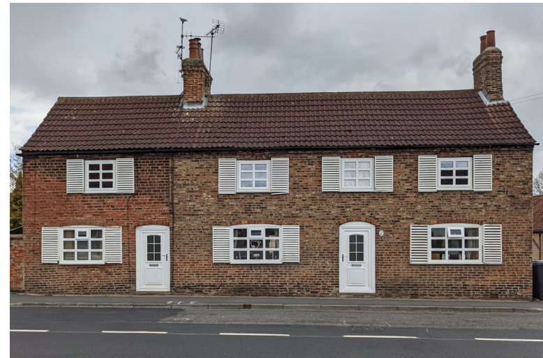
Number 49 main Street, a 19th century former farm house much altered with new reconstituted stone pantiles, uPVC windows and doors and shutters
