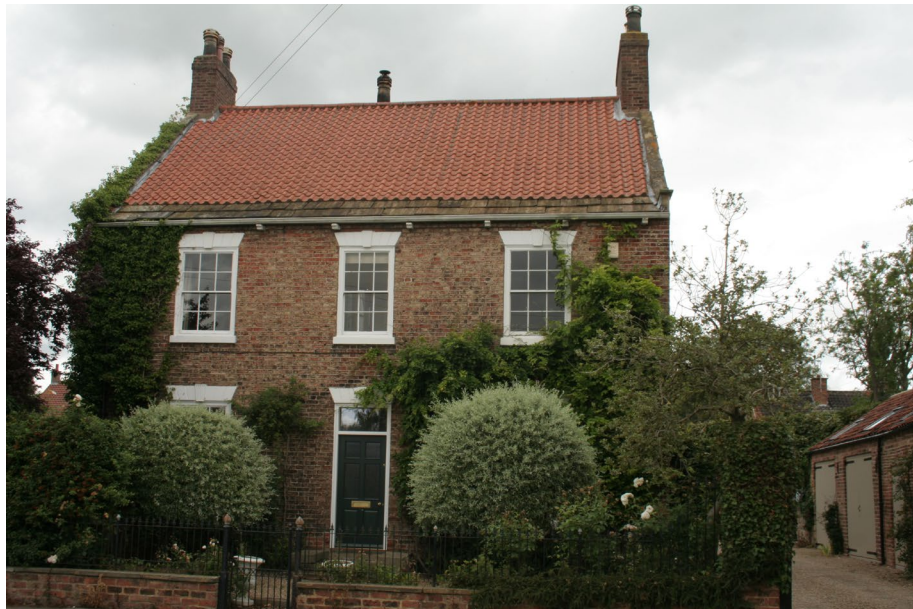
The Grade II listed Old Vicarage built in the late 18th century showing the building set back from the road with a low brick front wall and mature shrubs. Note that the clay pantiles have been replaced like for like and the yorkstone roof slates in the eaves have been retained. The windows and door are also replacements but reflect the historic proportions well.
