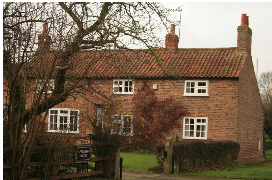
uPVC replacement windows on a non-designated historic property on Main Street
