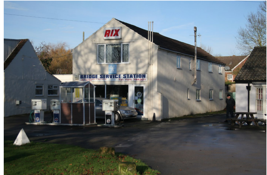
Landmark building, Bridge Service Station on Chapel Green
