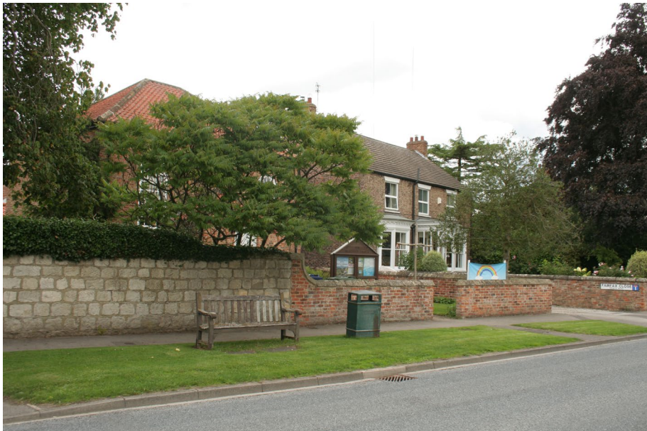
View of two boundary walls on Main Street, one in magnesian limestone and one in brick in front of the Grade II listed Wesleyan Methodist Chapel built in 1818
