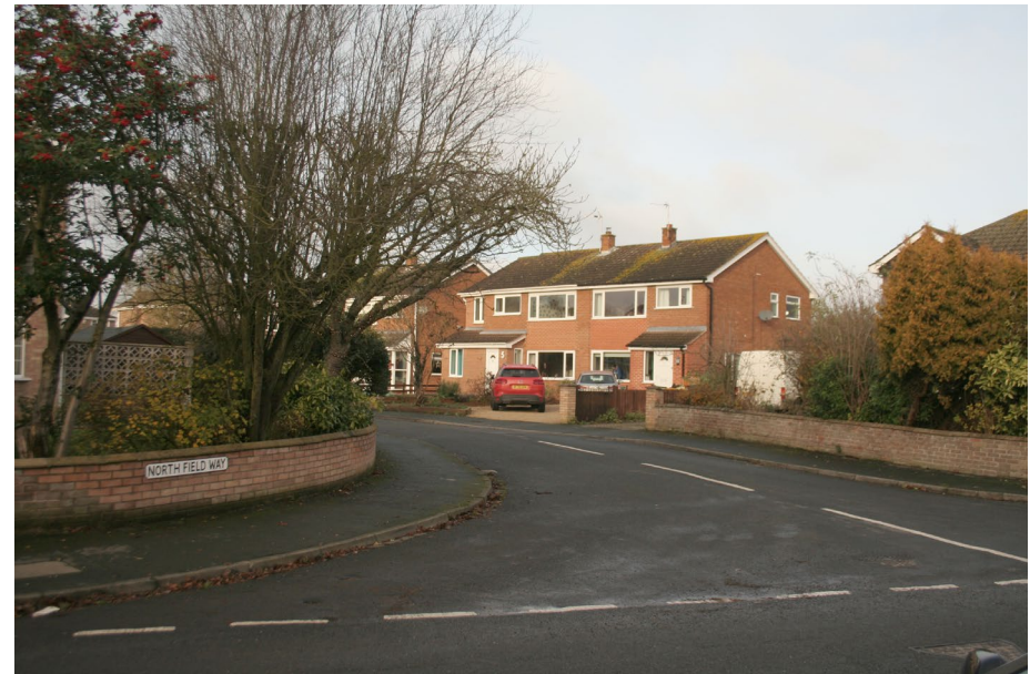
The junction of North Field Way and Main Street demonstrating the impact of standard late 20th century road design on character
