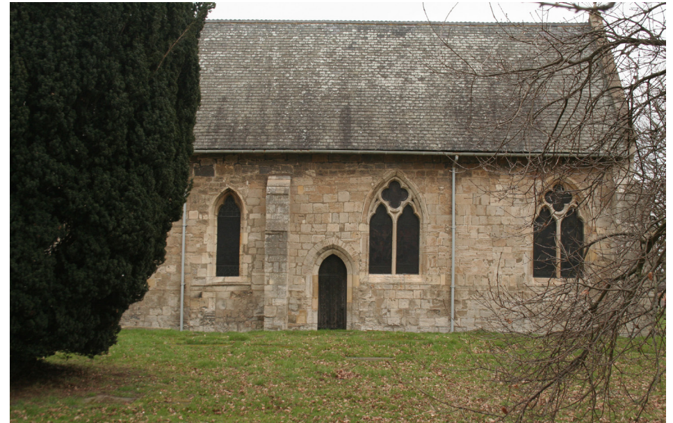
13th century door and 13th century lancet window to the left with later 14th century windows to the right. The whole elevation has been extensively restored in the 19th century
