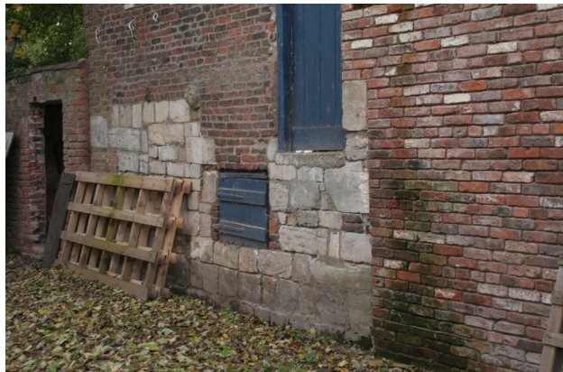
Example of possible medieval use of magnesian limestone and later hand made red brown brick off Sherburn Street
