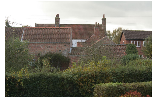
A view of the roofscape of properties on Thorpe Lane from Water Row showing traditional clay pantiles and the more recent reconstituted materials used on the late 20th century building on the right.
