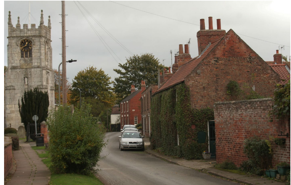
Former agricultural workers terrace opposite All Saints Church
