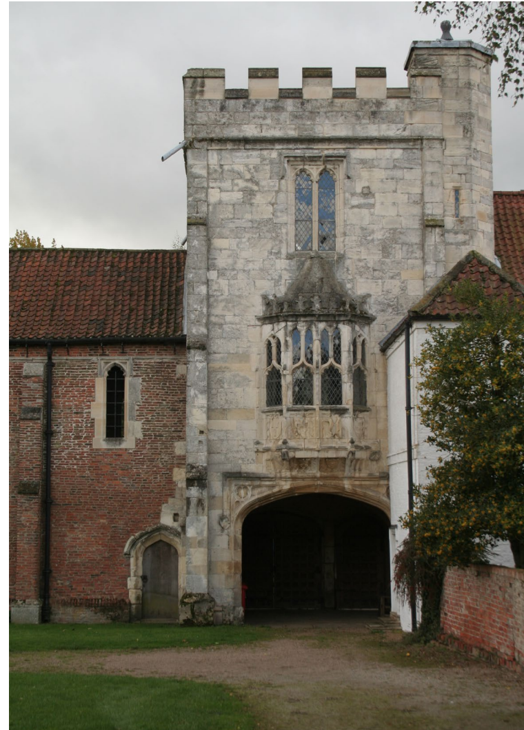
The Grade I listed early 15th century gatehouse to Cawood Castle taken from Thorpe Lane
