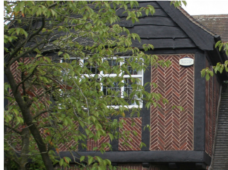
Detail of weatherboarding and herringbone brickwork on 20 Leeds Road
