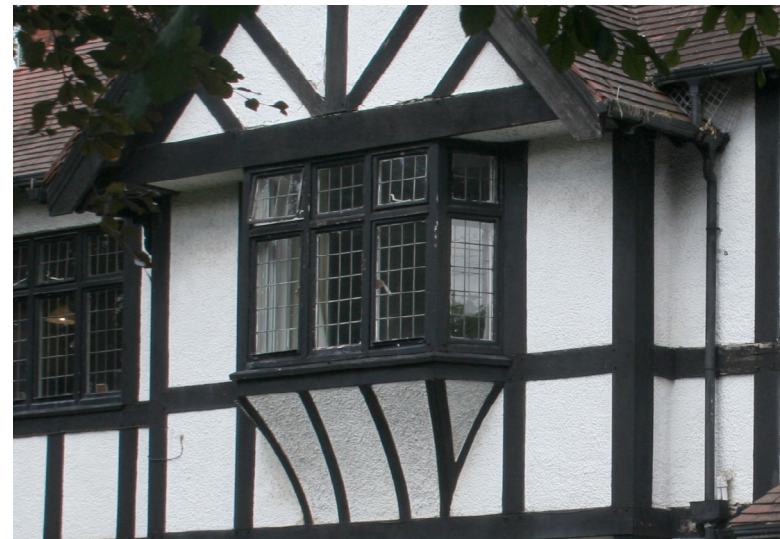
Detail of timber framing and oriel window on the Tudor House
