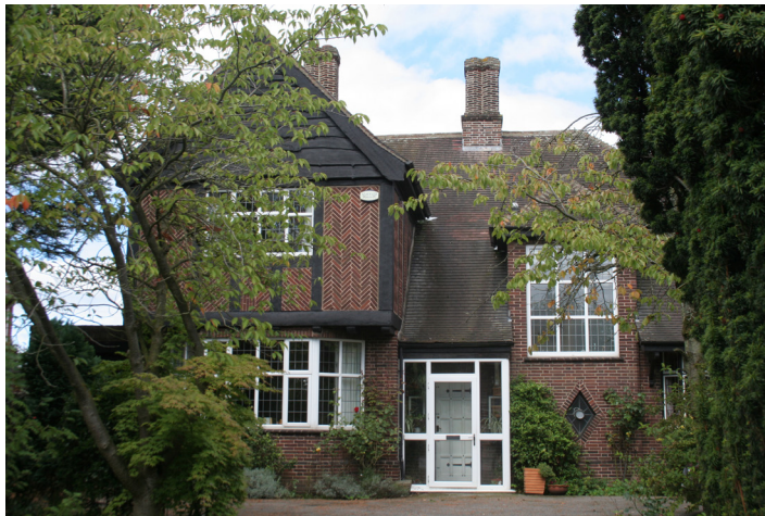
Detailing of number 20 Leeds Road showing timber framing, barge boards and brick work
