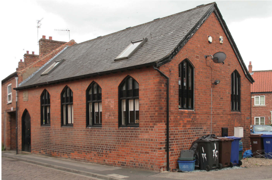
Rebuilt chapel on lower Millgate which is a landmark building
