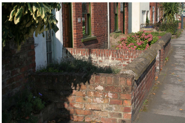
Set back properties behind boundary walls with small front gardens on Upper Millgate
