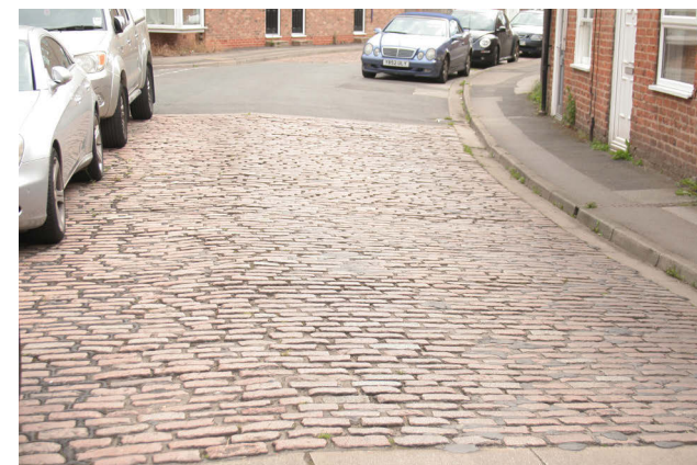
Use of Yorkstone setts as traffic calming measure and to break up the asphalt on Lower Millgate
