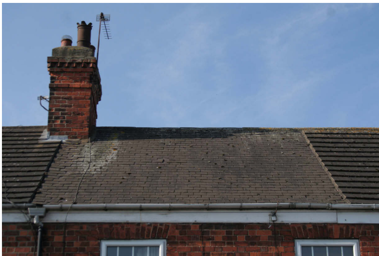
Traditional Welsh slate roof contrasting with modern reconstituted stone tiles to either side on Millgate
