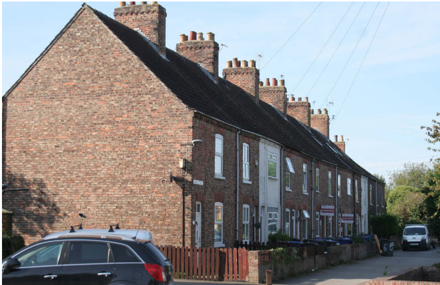
Annie Steet terrace in the Millgate conservation area and illustrating whole-sale refurbishment including a variety of uPVC window and door replacements as well as a new roof with reconstituted stone tiles
