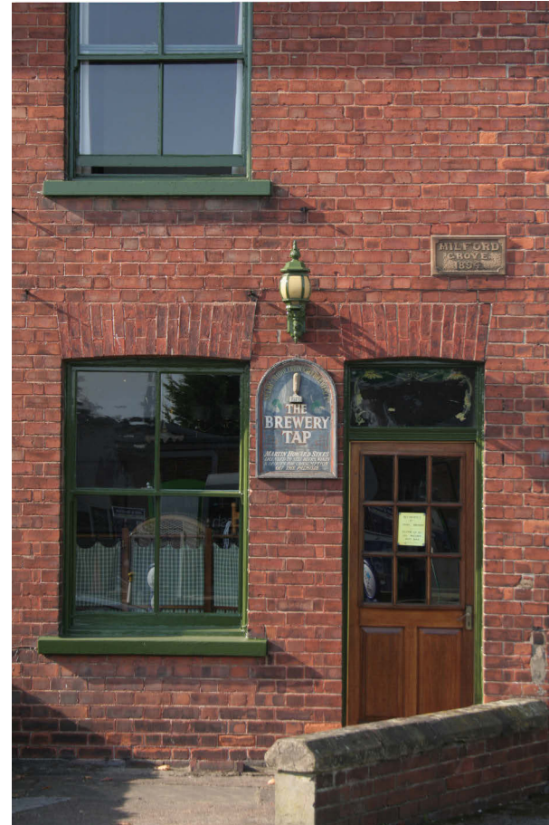
Well cared for traditional timber sashes at 131 Millgate
