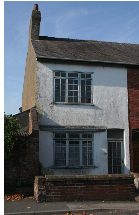
127 Millgate showing unusual timber windows with a ground floor bay all set back behind a boundary wall
