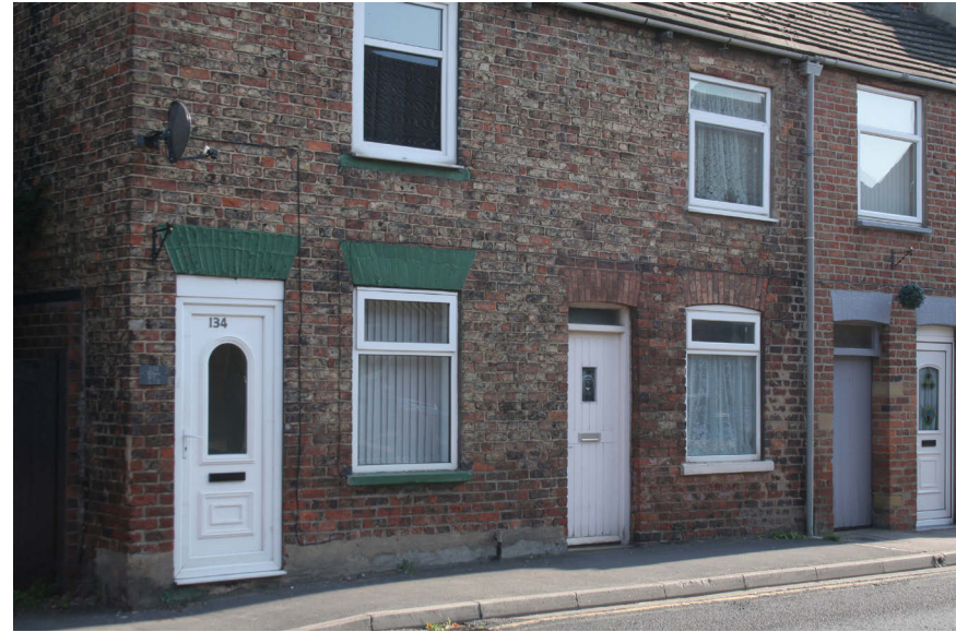
132 -134 Millgate with uPVC replacement windows and doors. The windows are top opening to compound the negative impact on historic character
