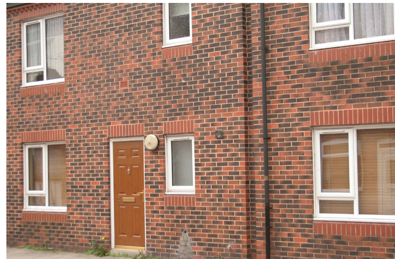
Firth Mews, although similar in form from the replaced 19th century terraces, demonstrates a departure from historic styles in the window and door detailing
