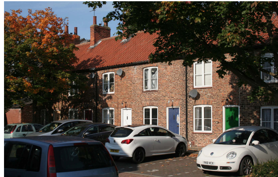
The Grade II listed Dobson's Row, showing replacement windows
