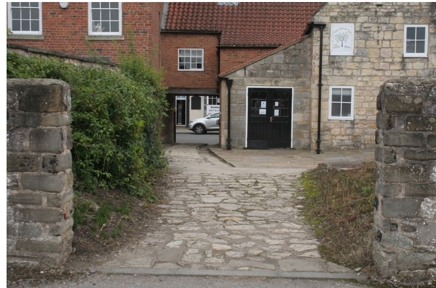
View of a side passage from High Street to the central area car park with traditional and original York stone setts and York stone slabs that are probably
