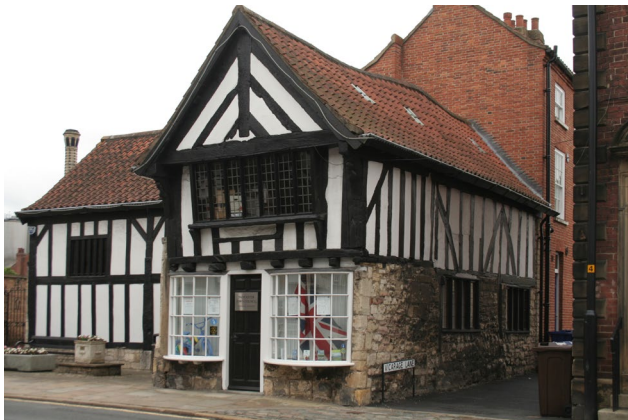
The timber framed Grade II listed 'Ark', 33 Kirkgate now the offices of the Town Council and other local community groups
