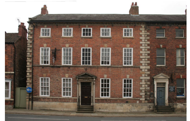
The listed Grade II Shann House, an 18th century residential property on Kirkgate (no. 47). Note the limestone ashlar footings, angle quoins and other decorative detail in brick and stone including the use of Flemish Bond in the main brick structure (more decorative than the more usual English Bond).
