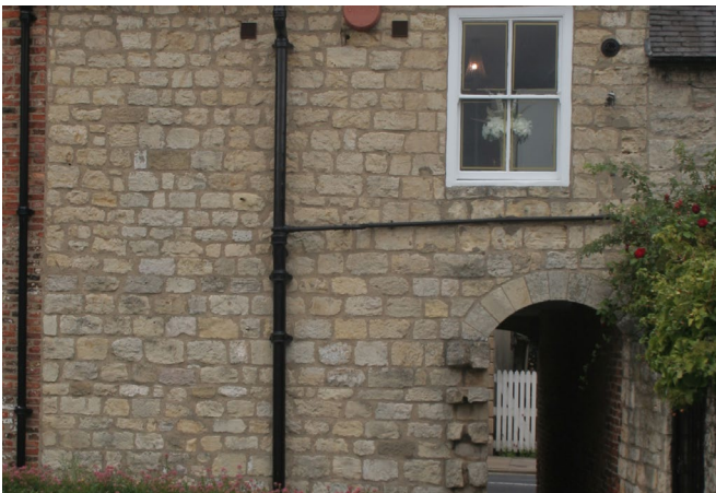
Example of rough hewn (not machine cut or sawn) magnesian limestone ashlar
