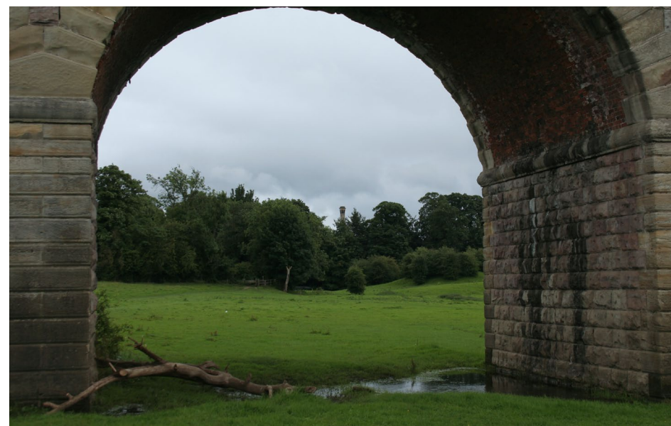
Contextual view 12. Looking through the former railway viaduct to the south
