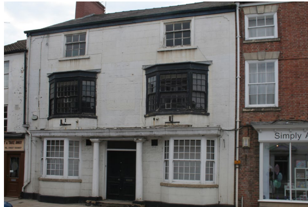
Ground and first floor projecting bow windows (18th century in date) on the High Street. Note the misaligned first floor bays which were a later addition
