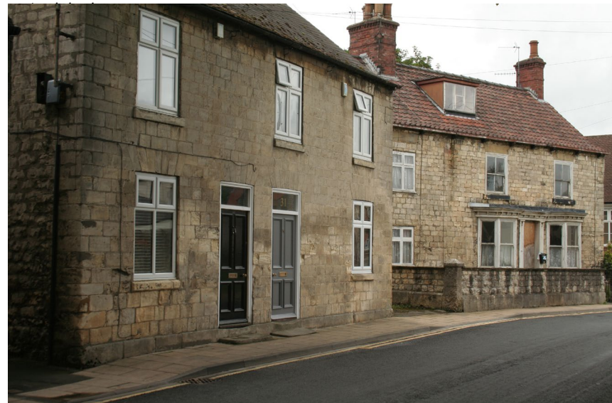
Late 18th and early 19th century cottage style terraces on Chapel Street with a mix of magnesian limestone ashlar and rubble construction
