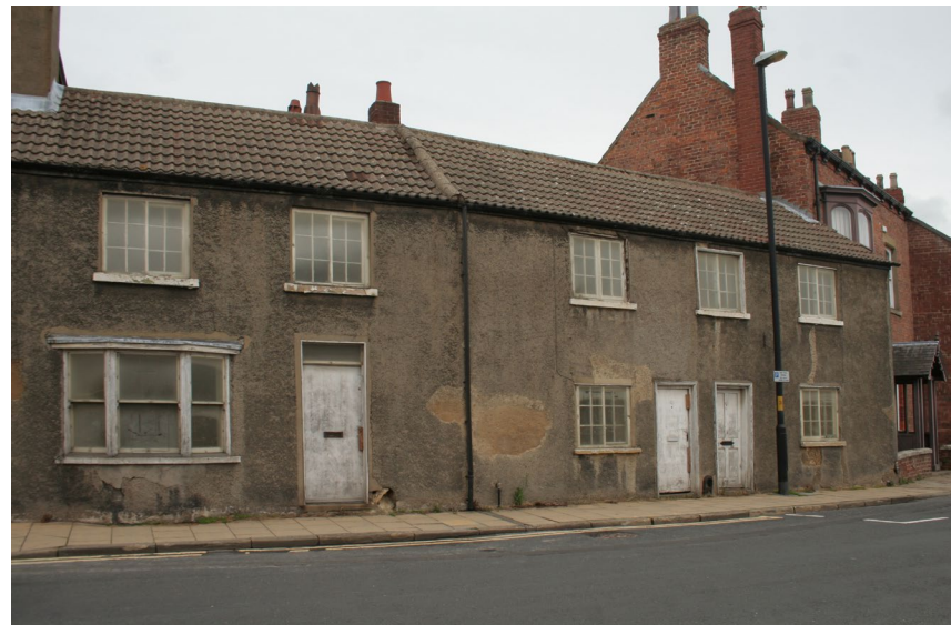
Rather dilapidated non-designated 19th century cottages on Westgate
