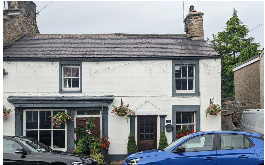
The grade II listed, "The Old Post Office". Note the restored and conserved traditional timber sashes and shop front
