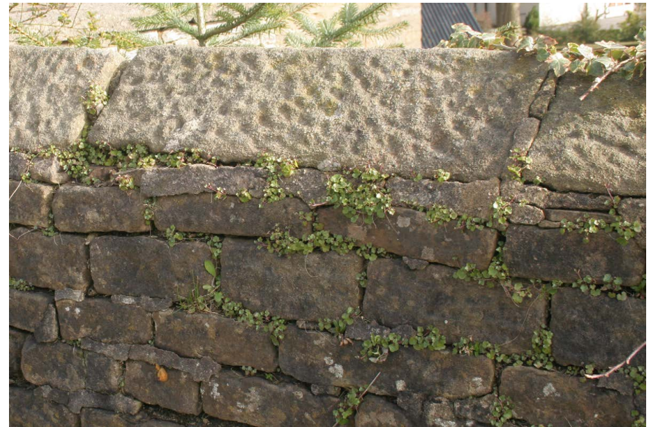
A typical boundary wall in Lothersdale. Note the tooled cap stones
