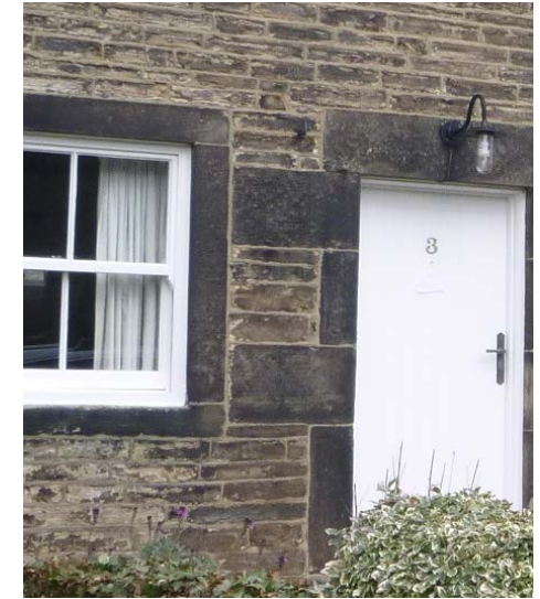
Millstone grit coursed stone on a building in Low Bradley
