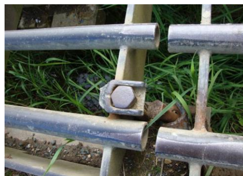
Longitudinal gap greater than 15mm
