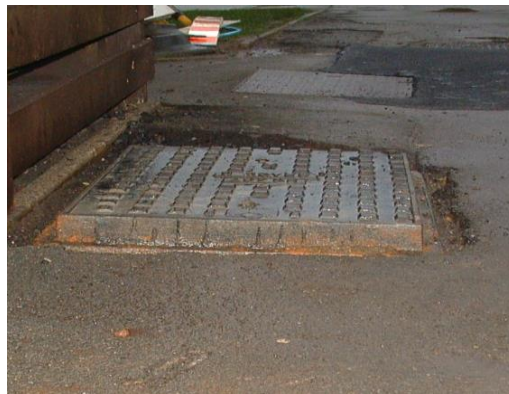
Protruding Inspection cover
