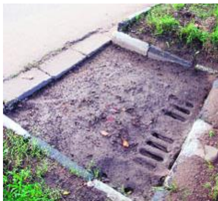
Gullies blocked by silt
