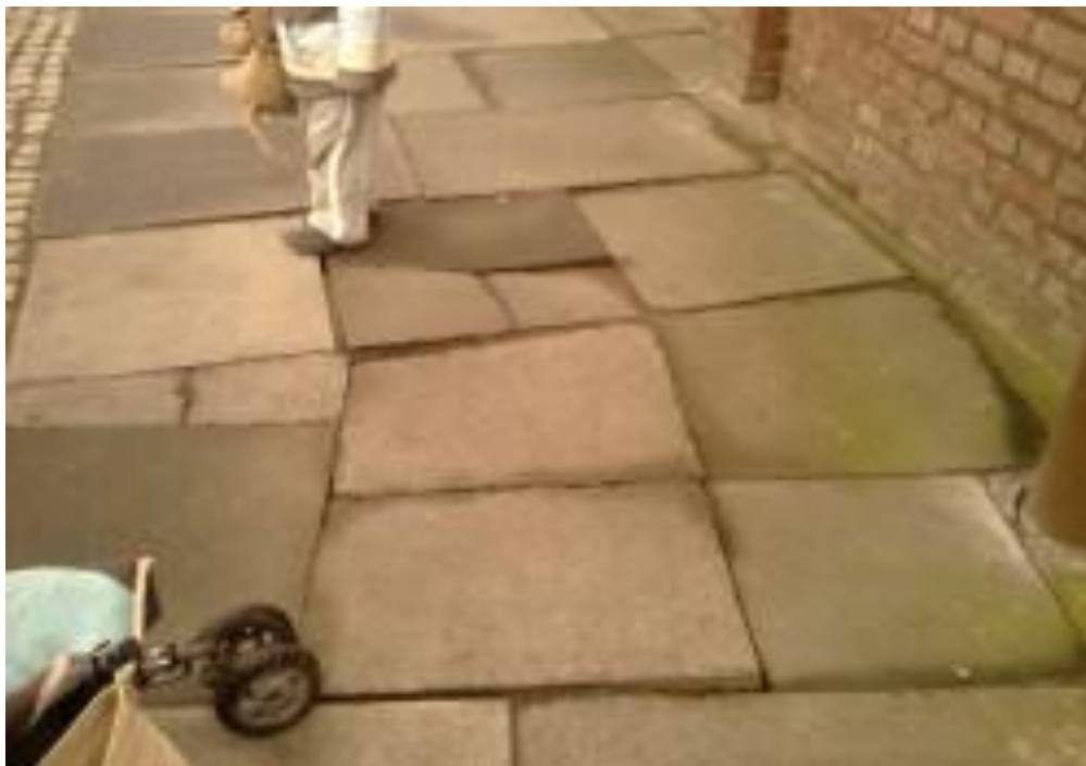
Loose paving stones
