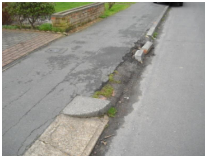
Kerb misaligned horizontally
