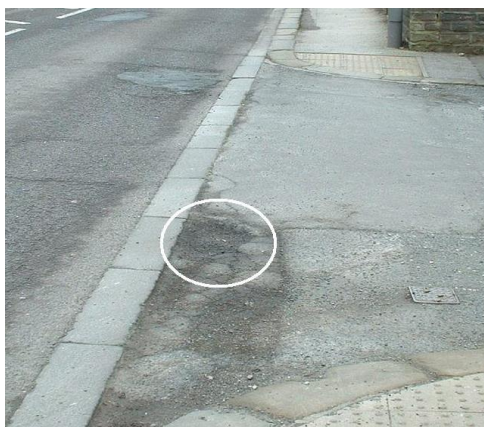
Potholes in pedestrian crossing of side road
