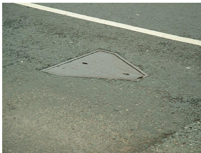
Worn and polished inspection cover
