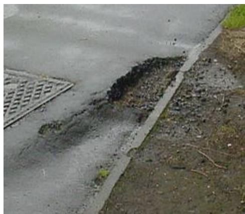
Pothole in footway exposing unbound material
