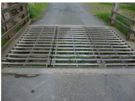
Longitudinal gap greater than 15mm
