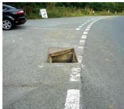
Missing Inspection cover
