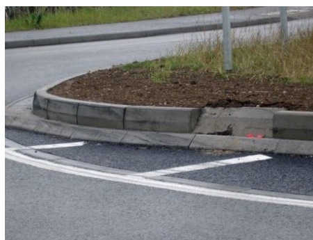
Kerb misaligned horizontally away from carriageway
