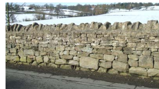
Wall opposite The Old School Room
