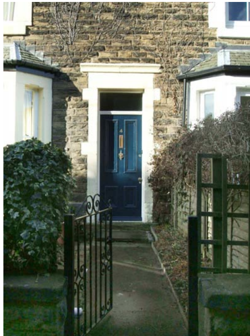
Door details at 4 Mill Lane
