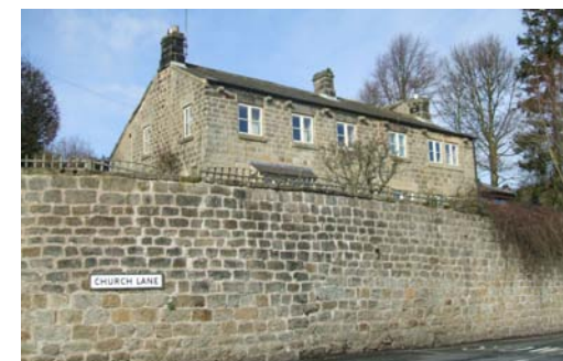
High retaining wall at Woodcock Hill
