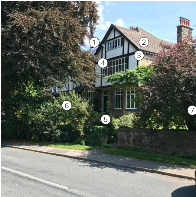
Photograph 10: Burn Bridge Road
