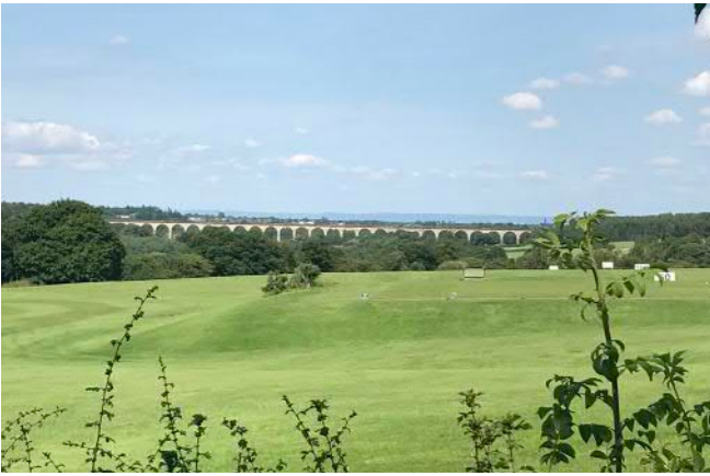
Grade II* Listed Crimple Valley Viaduct
