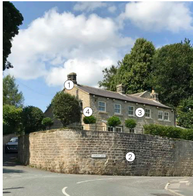
Photograph 14: Junction of Church Lane, Spring Lane and Main Street
