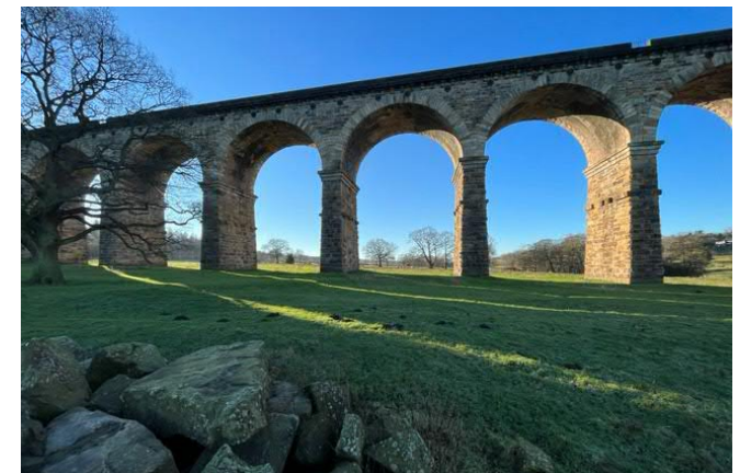
Crimple Valley Viaduct
