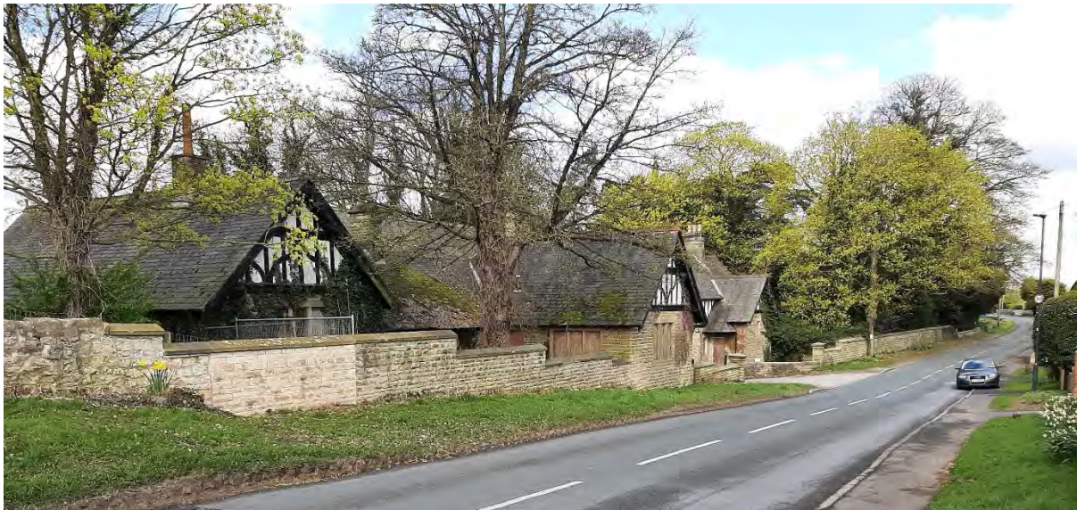
View 2 of outbuildings to the south of Fircroft and boundary wall running along Wighill Lane
