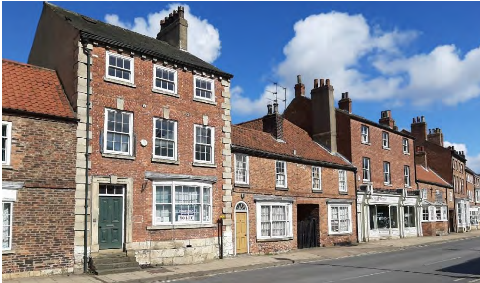
View of 28 High Street (to left) and 24 and 26 High Street (centre of photograph)
