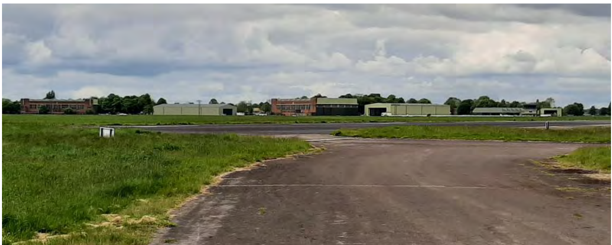
Above: Photo 5 showing aircraft hangars present in context with the airfield tracks.
