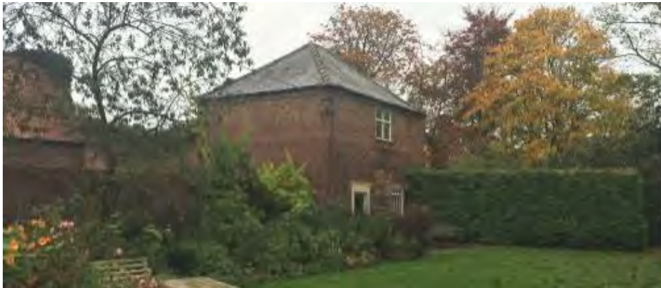
Above: Photo of Dovecote, south east elevation, from within the Hall's gardens – source: AAH Planning Consultants' Heritage Statement, October 2016 submitted with application 2016/1257/OUTM.
