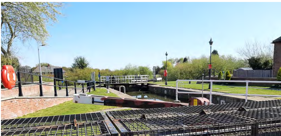
Above: View of the lock and lock gates from the south
