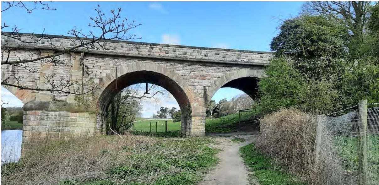
View of disused railway viaduct
