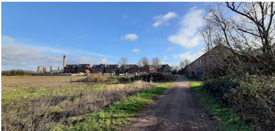
Above: View 4 - Looking east, along footpath – former farm buildings present to the right hand side.
