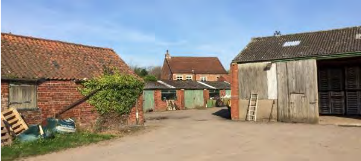
Above: Photo 2 - Farm buildings (Garth Lodge behind), Source: Archaeology & Built Heritage Assessment by Pegasus Group, dated May 2017 in relation to planning application 2017/0526/OUTM. Range of buildings to left date from 1845-8 or earlier. Those directly behind Garth Lodge dating from between 1845-8 and 1906.
