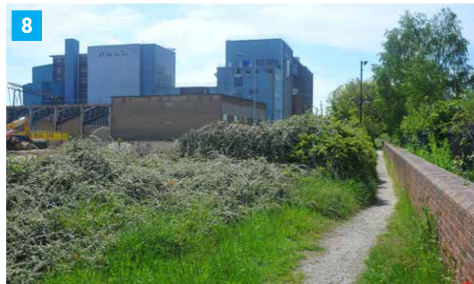
Former landscaped enhancement area requires maintenance refurbishment
