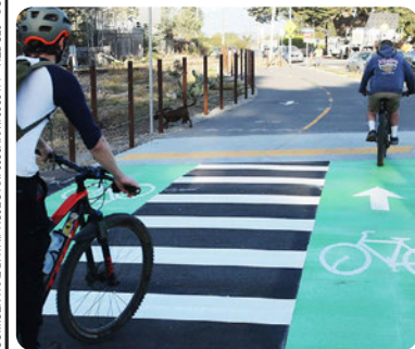
raised zebra crossing with consistent colour surface to promote branding of Cinder Track. Surface Colour red, orange or terracotta. Exact colour TBC at next stage
