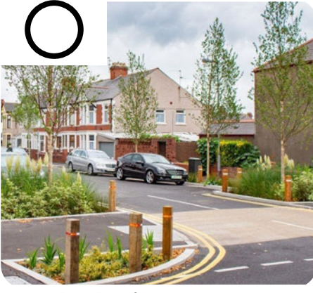
Speed reduction raised table with planted build outs to improve amenity.
