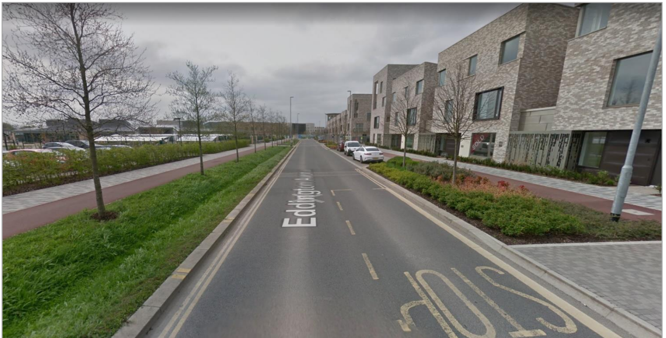
Figure 5-3 – Kerbed Cycle Track Separated from the Carriageway with SuDS Example
