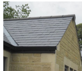
× Less appropriate man-made slate
