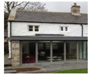
✓ zinc roof to extension (Austwick)
