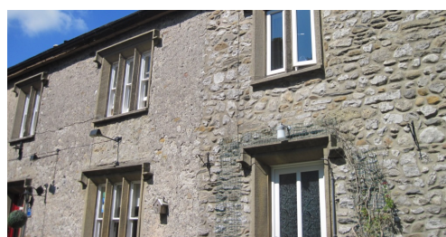
Left: lime roughcast render & sash window Right: rubble stonework & casement window
