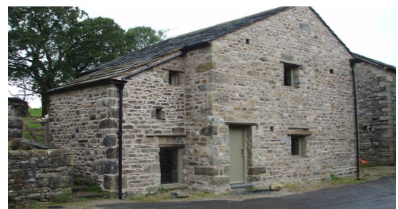
Windows set back with grey/green paint finish
