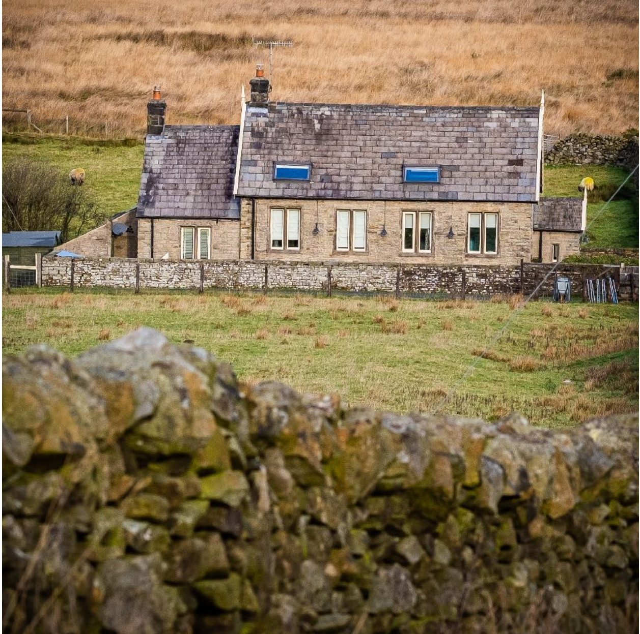
Brock A Bank, formerly Keasden Methodist chapel
