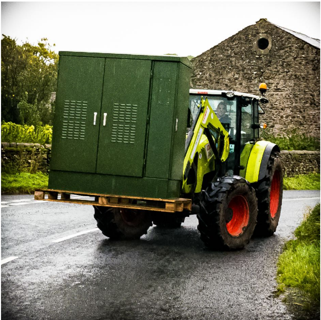
Delivering Clapham B4RN cabinet
