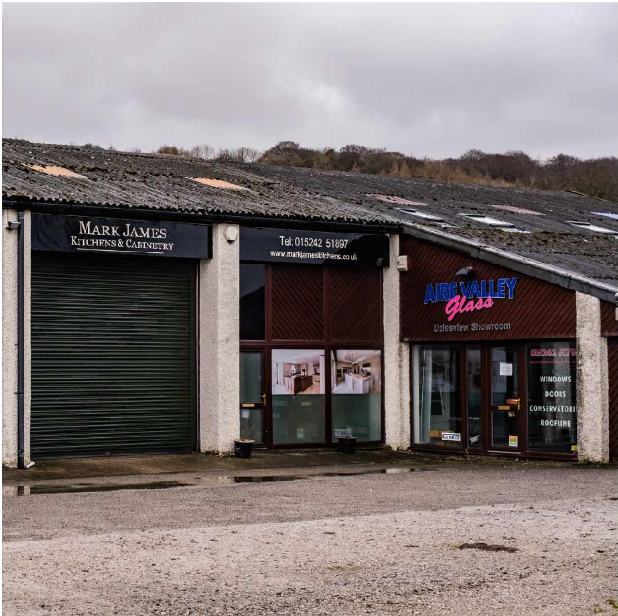
Aire Valley Glass and surrounding units, Clapham
