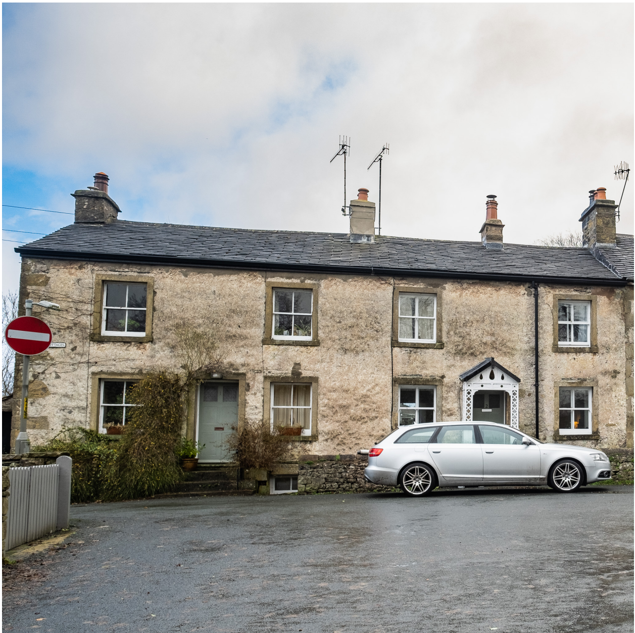
Vernacular cottages in Clapham let at an affordable rent by the Ingleborough Estate
