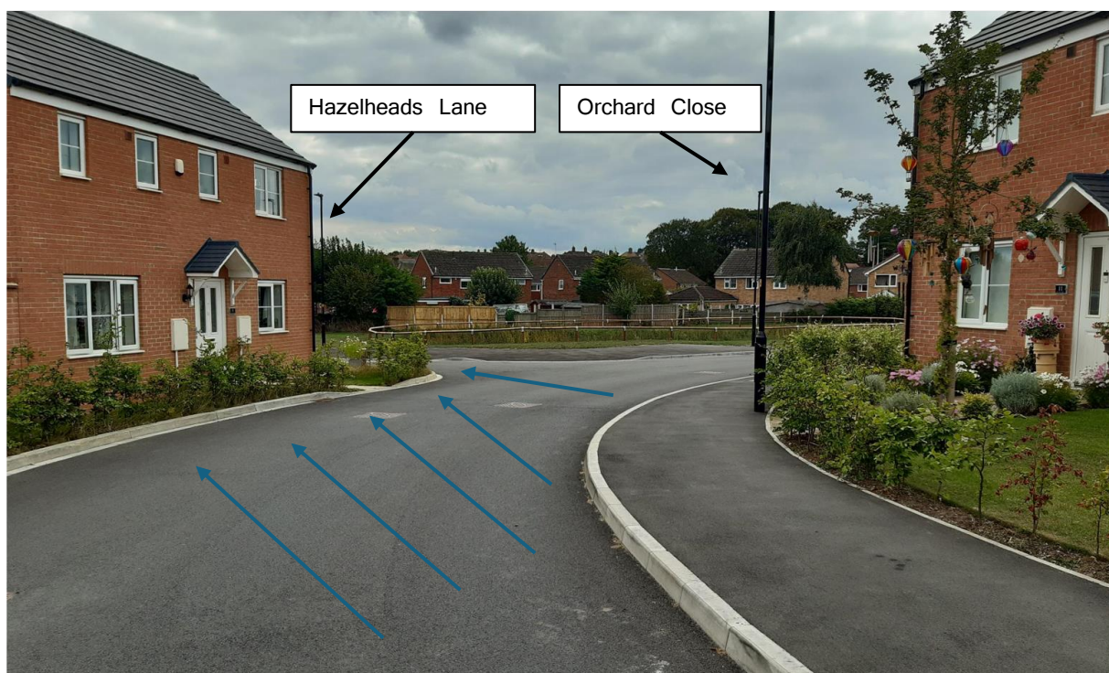
Figure 11: Carriageway Crossfall Bramley Way
