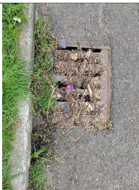
Figure 9: "Blinded" Gully on Blind Lane
