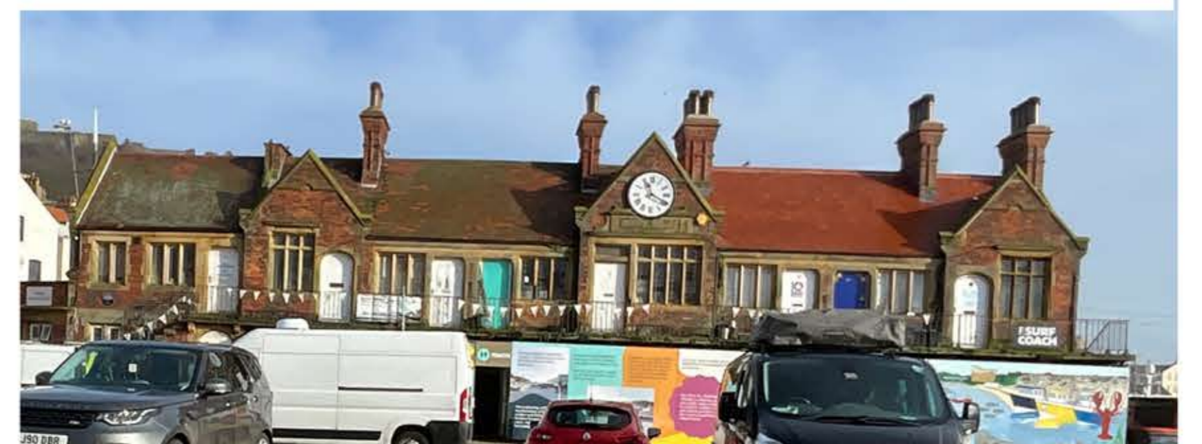
Image - North West View of Building 1 (Google Maps)
