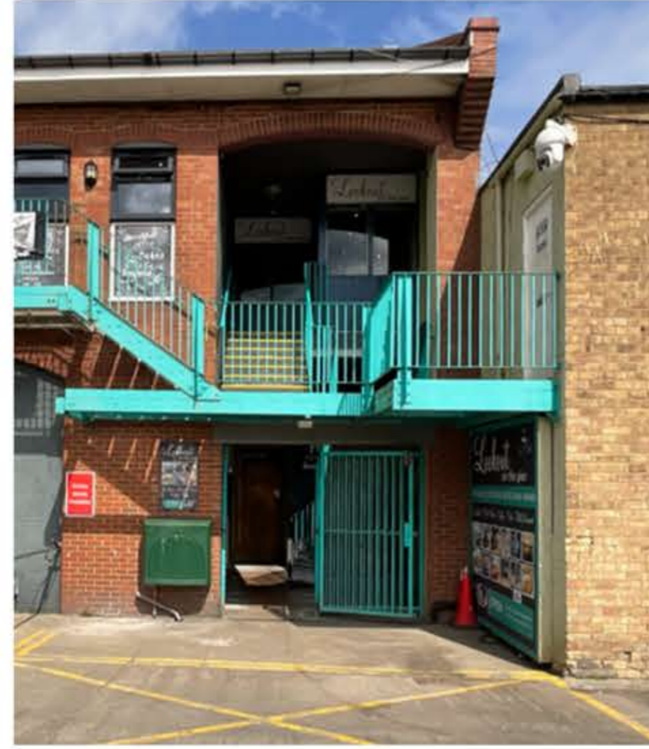
Building 3 existing stairs/ entrance
