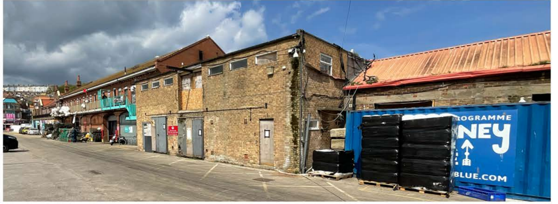
Existing location for Building 4
