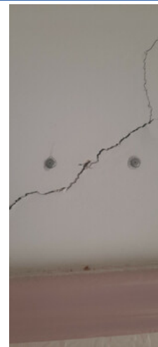
Internal front bedroom right hand side party wall - Visit #8
