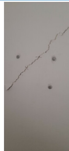
Internal right hand side party wall - Visit #8
