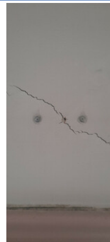
Internal front bedroom external wall left of window - Visit #8
