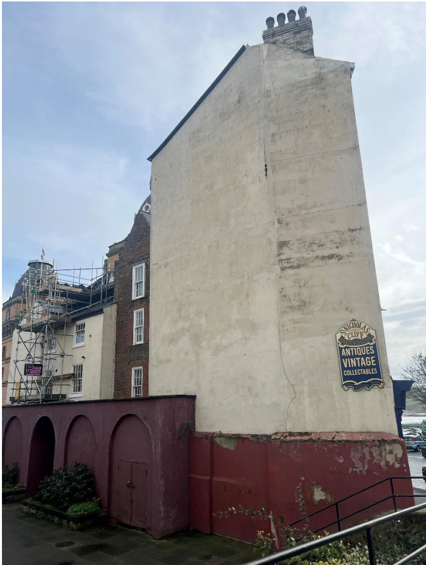
Figure 5 – Elevation view from pedestrian footpath at St Nicholas Cliff
