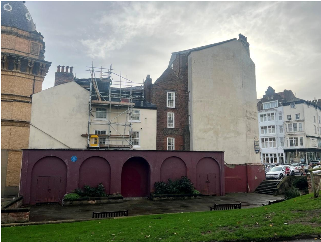
Image taken from the footpath on St Nicholas Street, showing the primary elevation - white gable end wall to the right of the image and the secondary elevation – the burgundy single storey wall shown across the centre left of the photograph.
