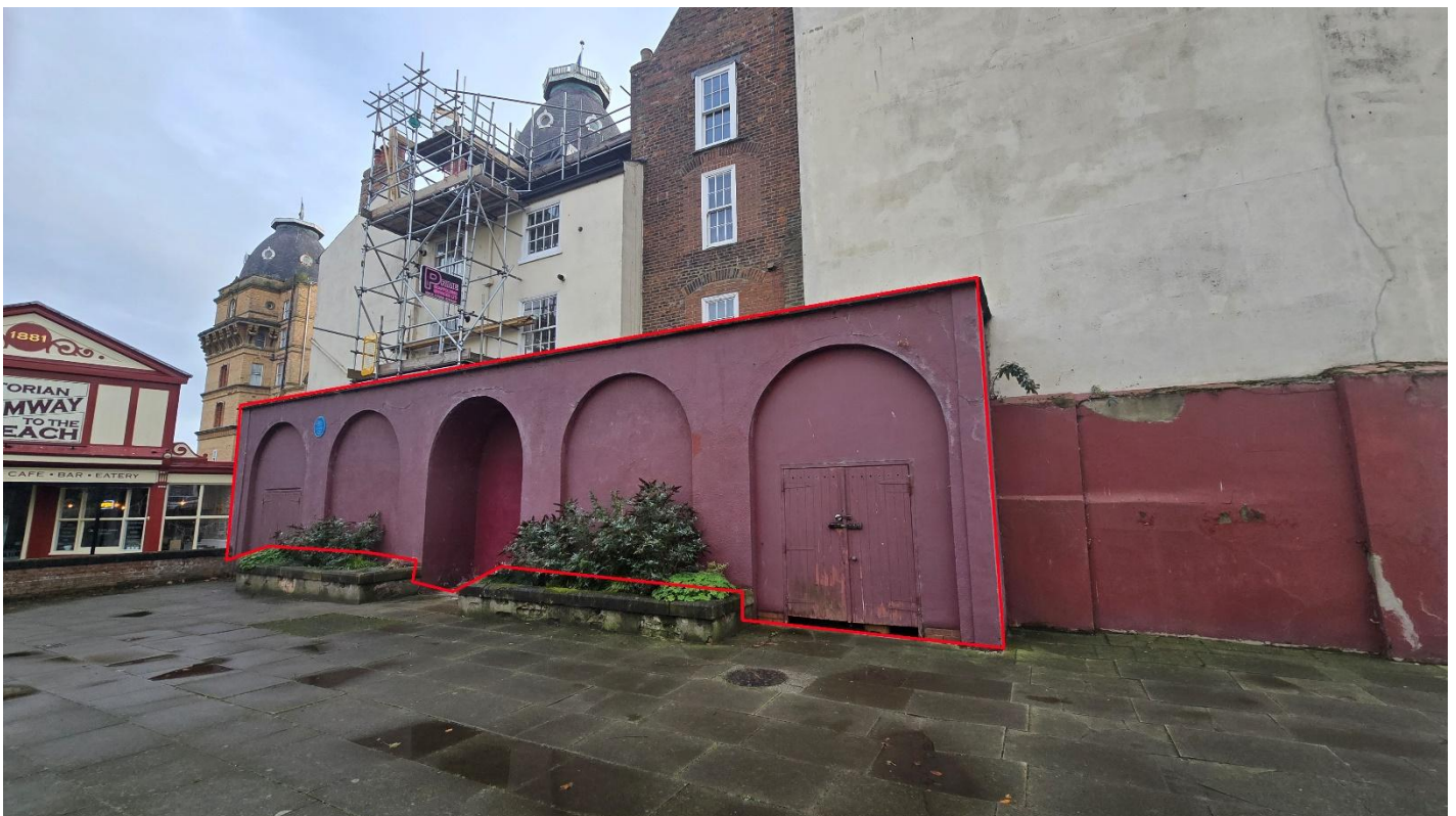
Figure 4 – Adjacent wall identified as an element for consideration in the design proposal
