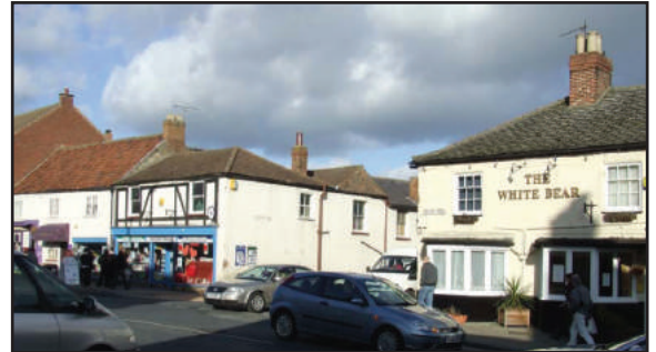
Figure 29: Intersection between Market Place, South End, Bridge Street and Sussex Street.
