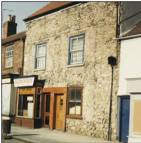
Figure 8: 21 North End cobblestone under render
