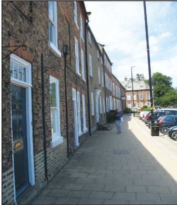
Figure 6: Buildings on the west side of North End
