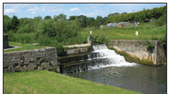
Figure 20: The Harbour and Weir.
