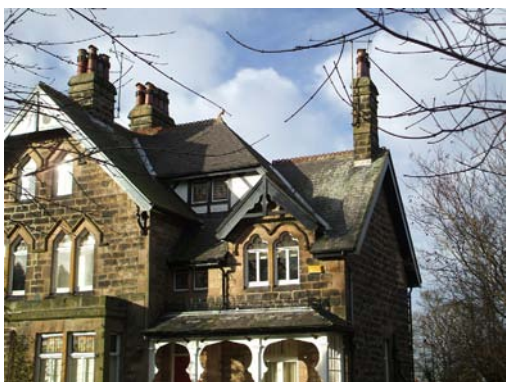
Complex roof forms with ornate barge boards and tall chimneys. Victorian Gothic windowheads and covered porch with timber posts and a projecting stone bay.
