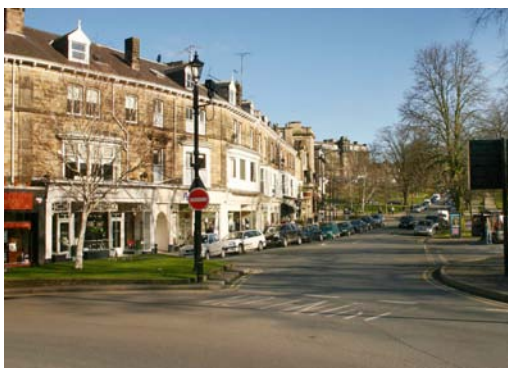
The use of stone walling and slate roofs predominate.
