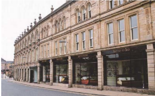
2-24 Crescent Gardens, known as The Grosvenor Building, have retained many of their original elegant shopfronts.
