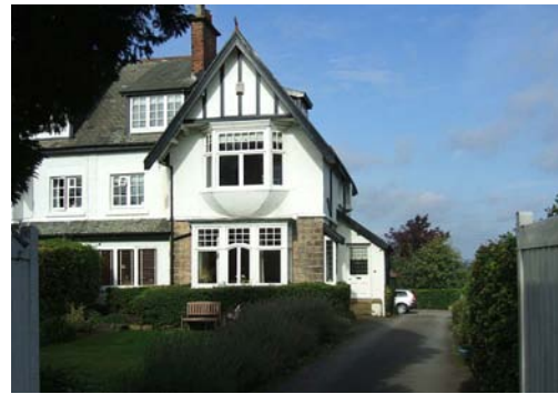
The use of render at first floor with half timbers effect above. Feature oriel window above three light window with heavy timber mullions and small paned upper sashes. This example from the Duchy estate.
