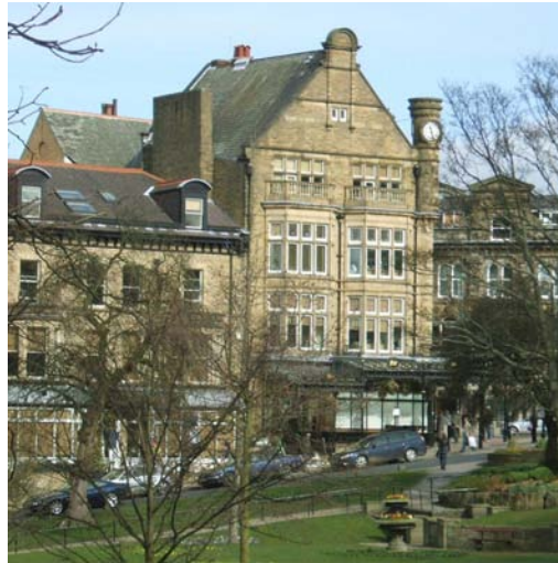
Welsh slate roofs have a 'heather' colour and are often used with contrasting clay ridge tiles. The higher roof (Betty's) is green Westmoreland slate.
