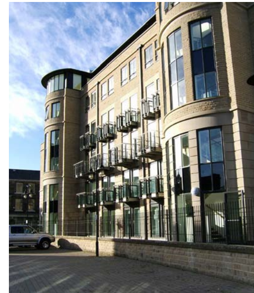
The demolition of the Western Block of the Royal Baths enabled the construction of this apartment block.
