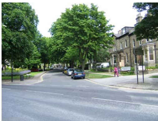
Alexandra Road (from Kings Road) Generous stone buildings exhibiting high quality detail.
