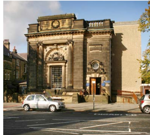
Carnegie Library on Victoria Avenue, part of an unfinished 'municipal palace' - the unbuilt section became Library Gardens fronting Station Parade.
