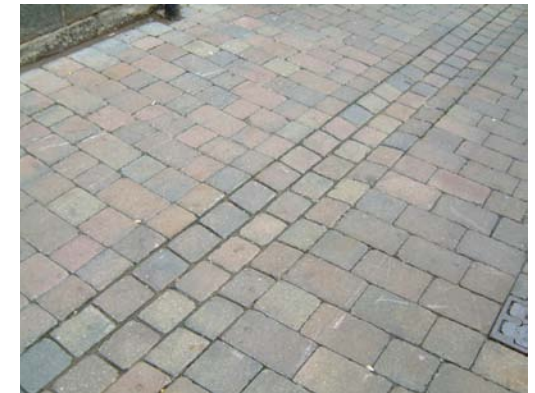
Paving detail on John Street, also pedestrianised.
