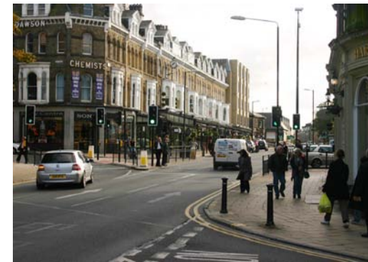
Prince Albert Row on Station Parade - a generous three storey height terrace with rooms in the roof.
