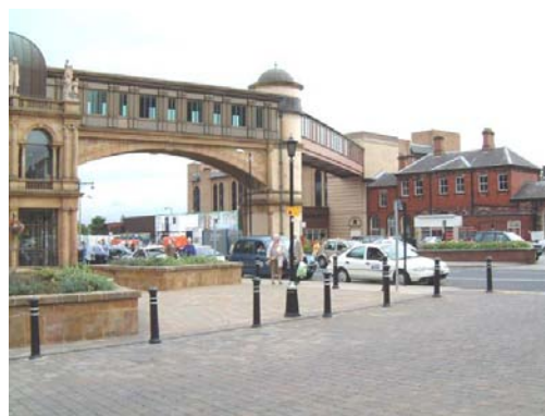
Bridge over Station Parade from Victoria Centre to Victoria Car Park
