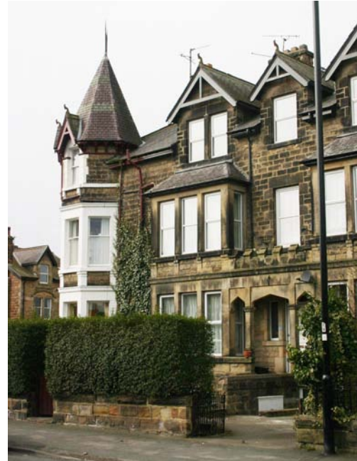
Buildings on Kings Road with turret at corner, dormers with decorative bargeboards with collars, two storey bay, mullioned vertical sliding sash windows.
