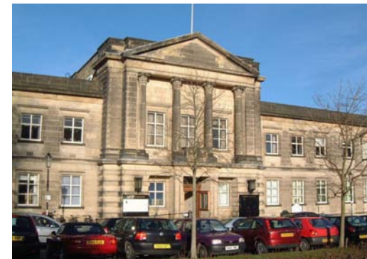
Council Offices facade on Crescent Gardens.
