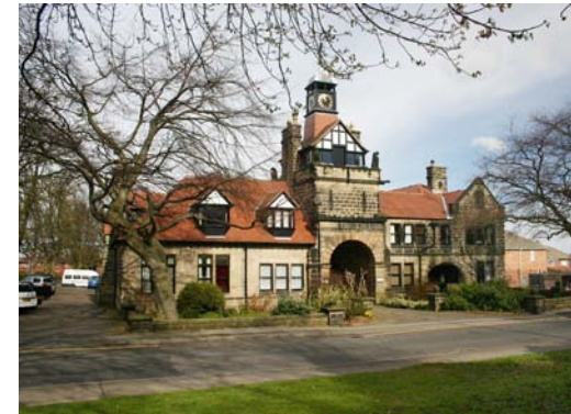
Grove House Stables, unusually roofed in red tile.
