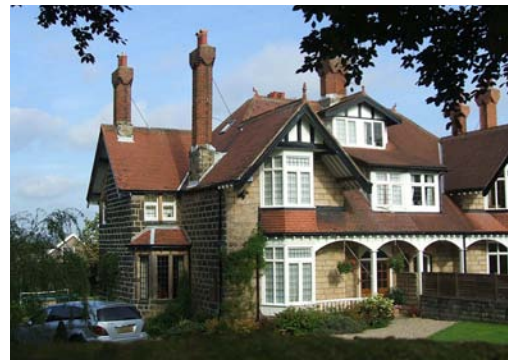
Again in the Duchy estate - small Rosemary tile on the roof and bays. Note the low eaves and the tall, narrow chimneys.
