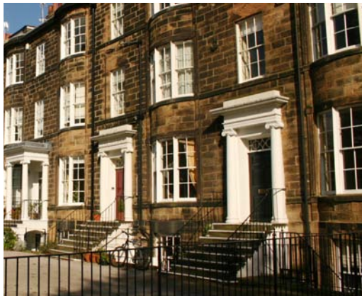
Multi-pane sash windows and classical doorcase in the Georgian manner seen on West Park.
