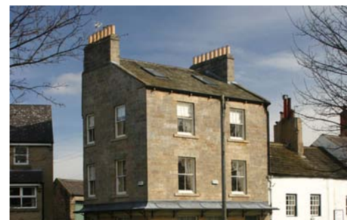
Two over two paned window, most are Victorian although some are of later construction.
