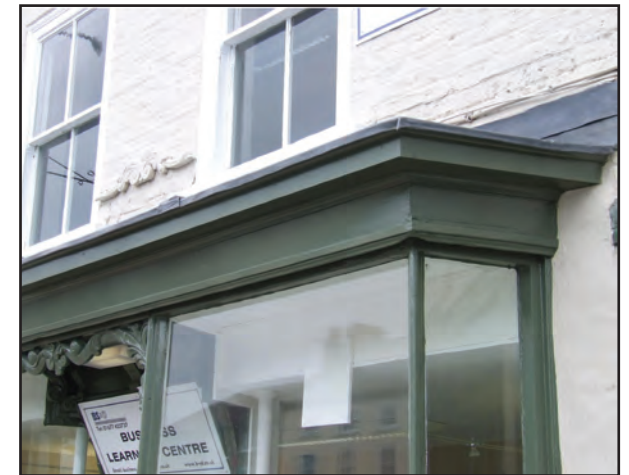
Figure 8: Projecting timber bay with shallow fascia.
