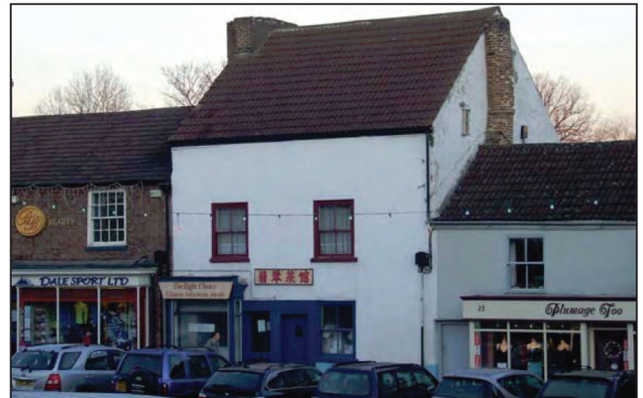
Figure 26: Poor selection of colours for the shop front, windows and render.
