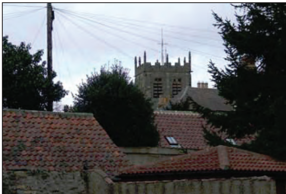
Figure 17: Clay pantile roofs.
