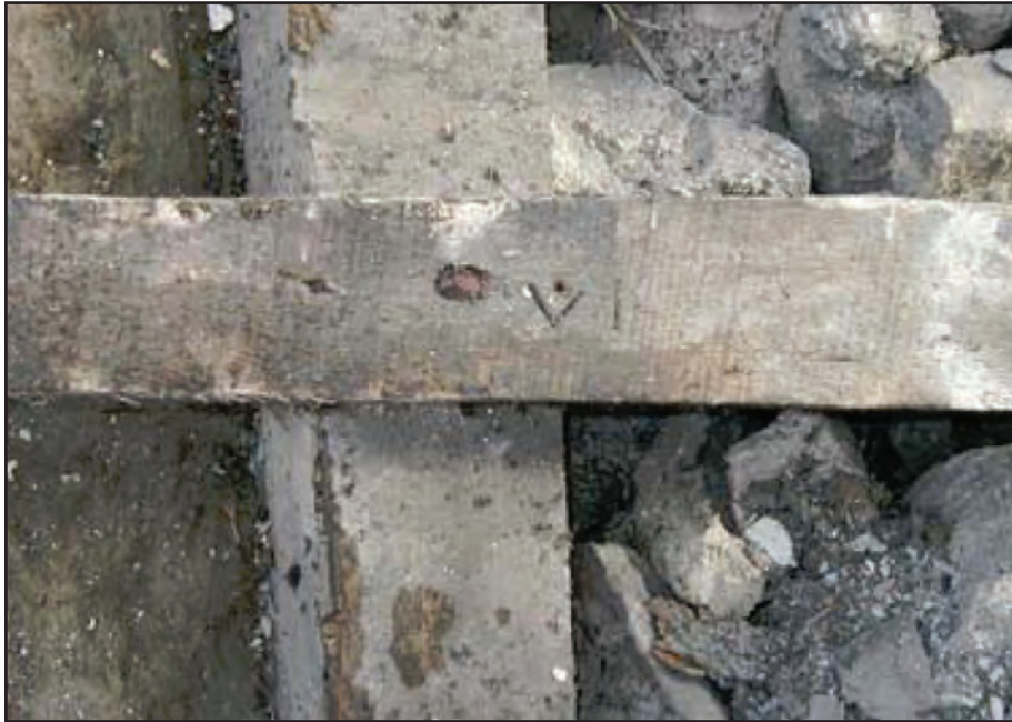
Figure 25: Carpenter's marks and other historic details should be saved.
