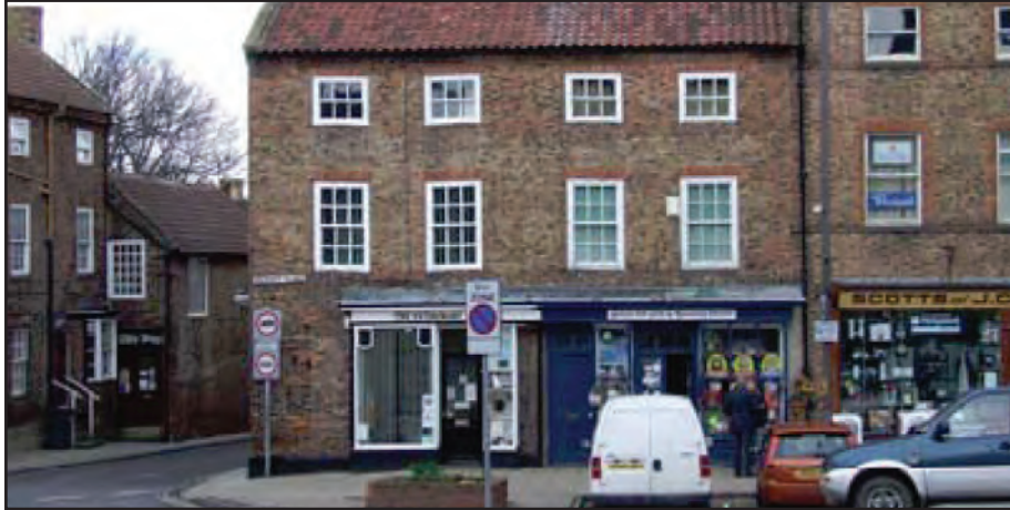
Figure 23: Traditional multi-pane sash windows with exposed boxing to early Georgian façade.
