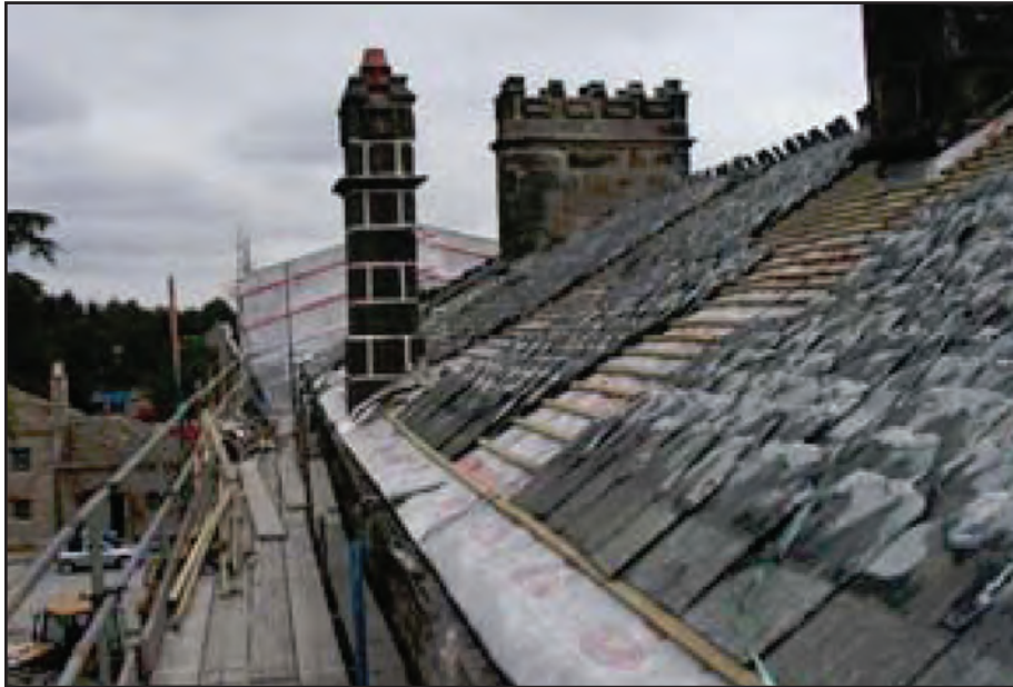
Figure 18: Slates stacked in diminishing size ready for laying.
