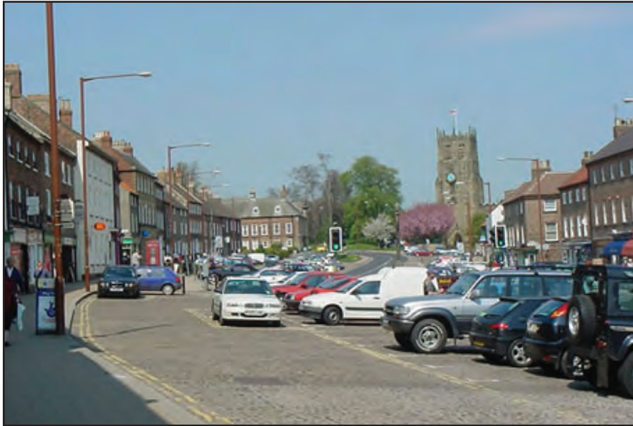
Figure 30: Historic cobble surface is a feature of the central core of Hambleton's market towns.
