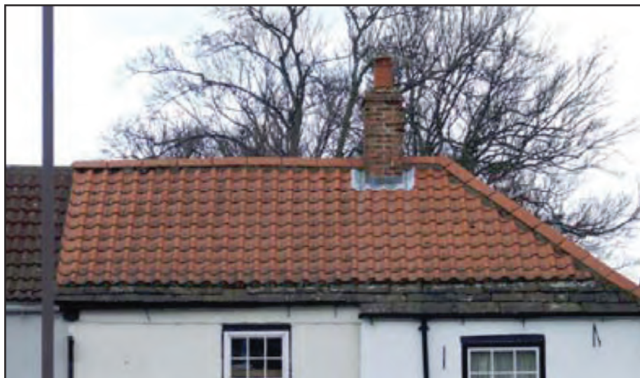
Figure 15: A traditional clay pantile roof with Stone Slate eaves course
