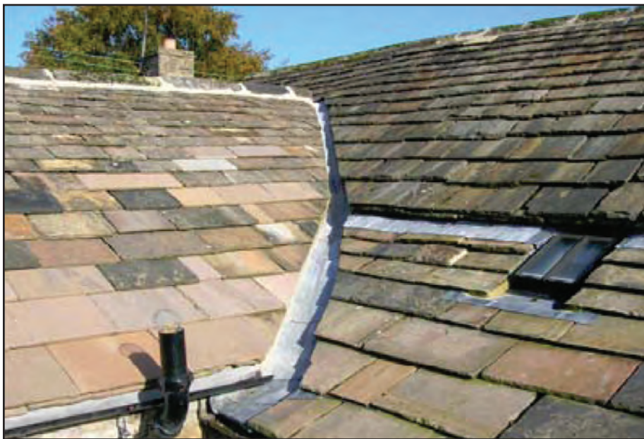
Figure 16: A well maintained stone slate roof.
