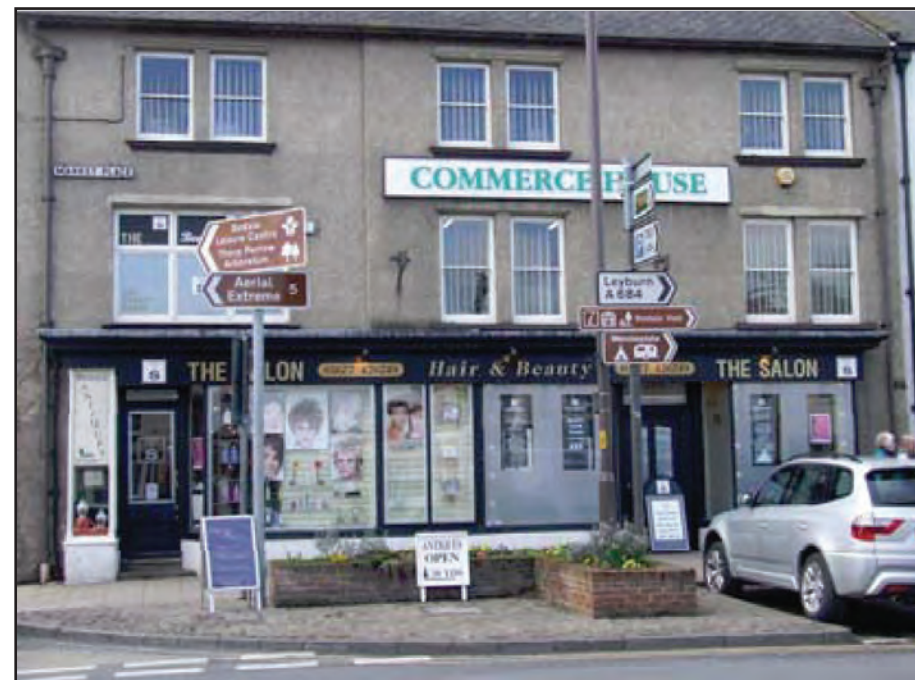
Figure 31: Over provision and poor siting of traffic signs.
