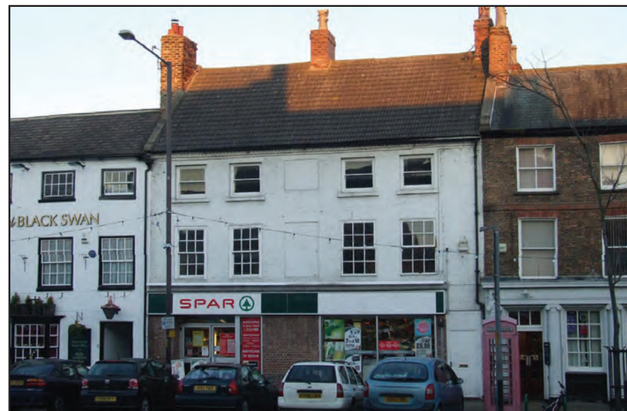
Figure 4: This modern shop front has no visual relationship with the upper floors.
