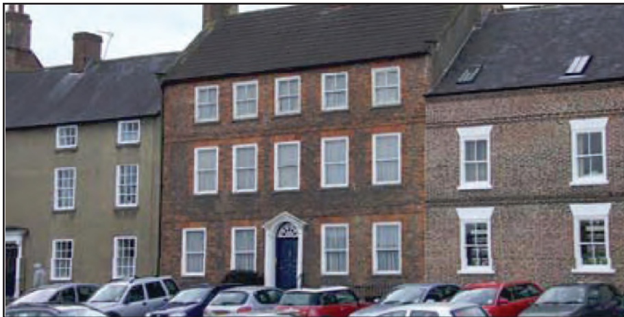
Figure 24: Fine Georgian façade spoilt by poor fenestration
