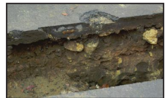
Cobbled surface under tarmac
