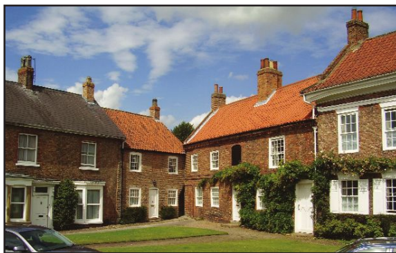
Houses to north east of Market Place
