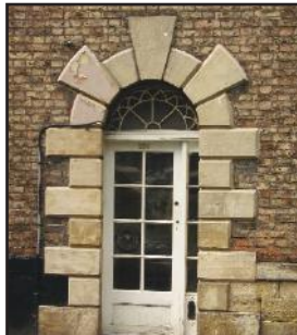
Quoined basket arched doorway
