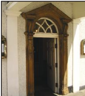
Stone pedimented door surround
