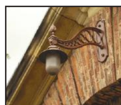
Former Police Station lighting
