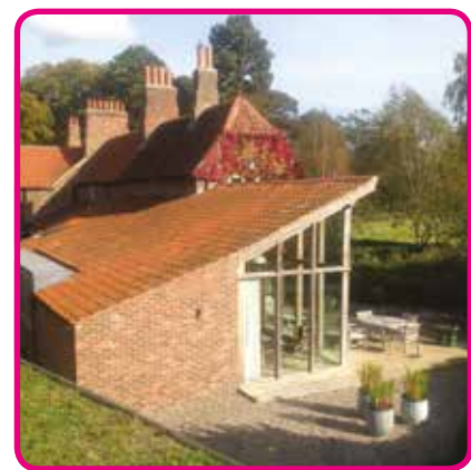
Fig 12: Modern extension at Midsummer Cottage uses local handmade brick and Incorporates a structural oak frame.
