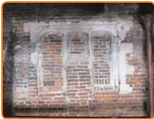
Fig 7: Fragments of mid 1500's high status fabric surviving within a modern barn at Rooper Hill
