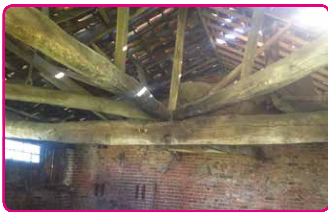
Fig 11: Oak roof at the Horse Engine House, Village Farm
